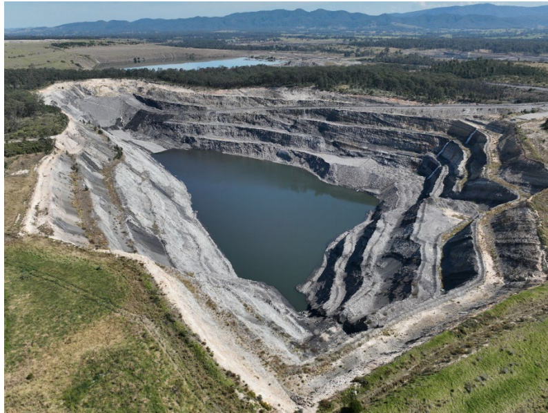
Plate 1: Avon North Pit Water Storage, looking south September 2024
