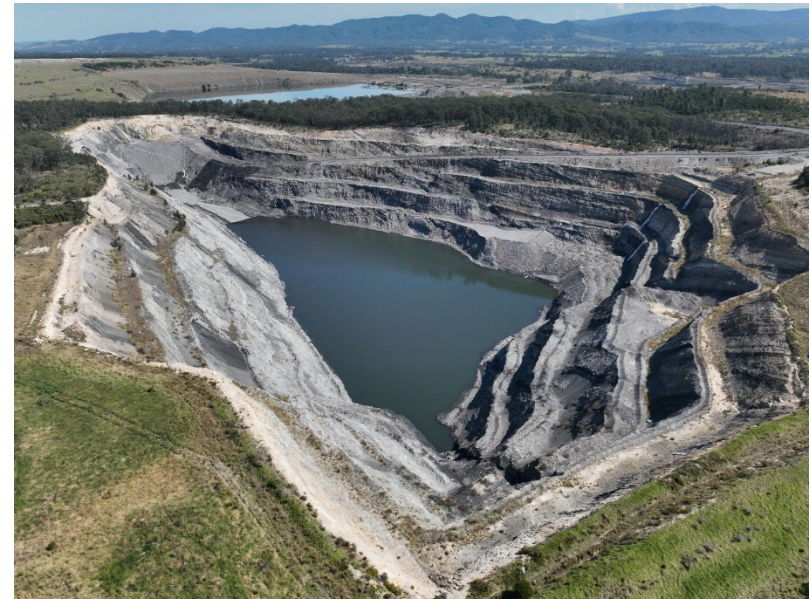
Plate 2: Avon North Pit Water Storage, September 2024.
