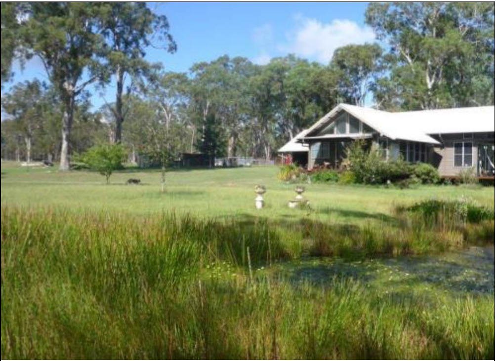
Plate 2 Survey unit 1 showing dam, house and associated buildings
