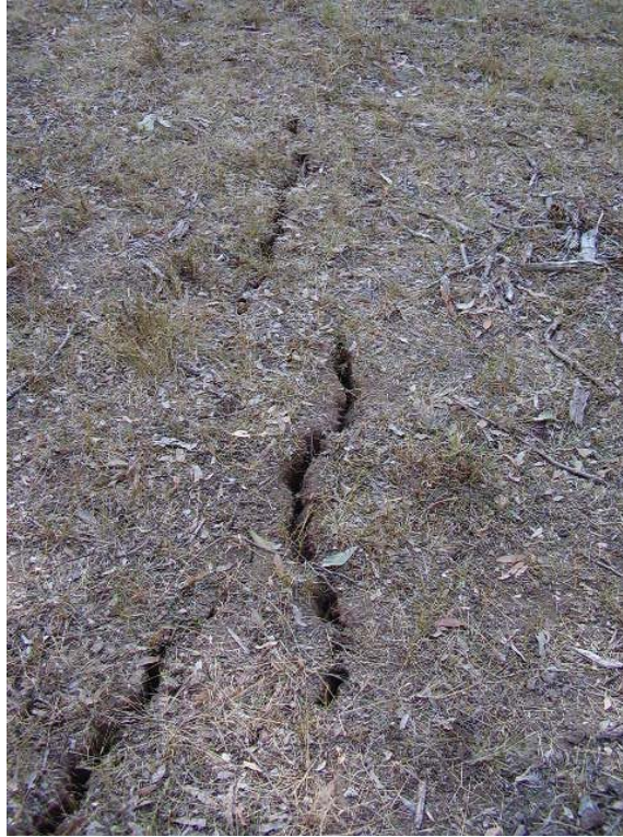
Fig. 4.5 Example of surface tensile cracking in the natural ground surface (observed in the Southern Coalfield at a similar depth of cover as in the Study Area)
