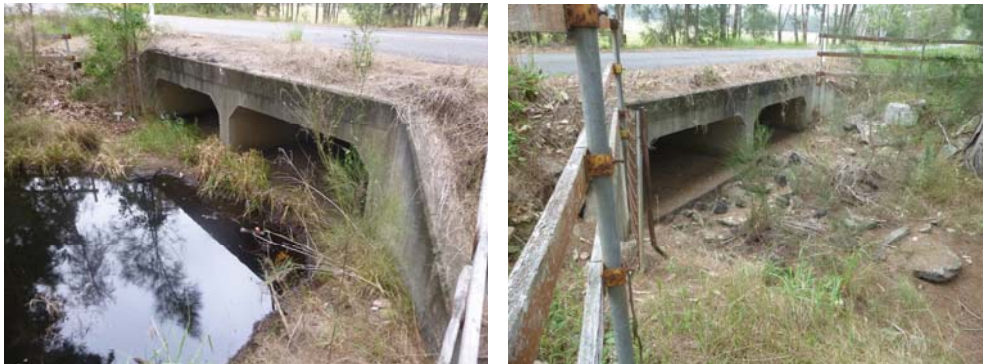
Fig. 6.2 Box culverts SCR-C1 (left side) and SCR-C2 (Right)
