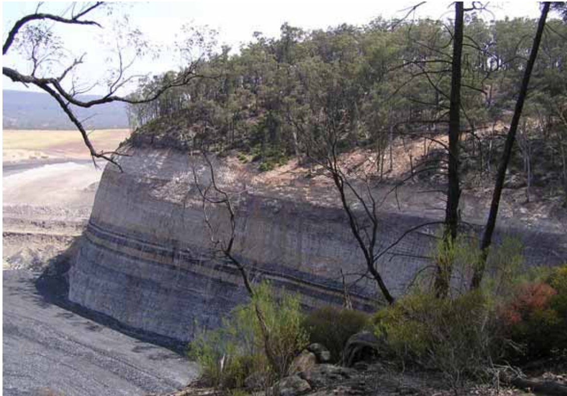
Plate 5: View north-west to Survey Area 25 (moderate simple slope) in OC1 Extension Area, bordering existing Open Cut 1 pit.
