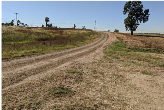
Track maintenance completed
