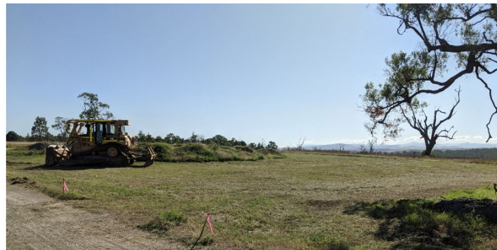
Gravel pad underway
