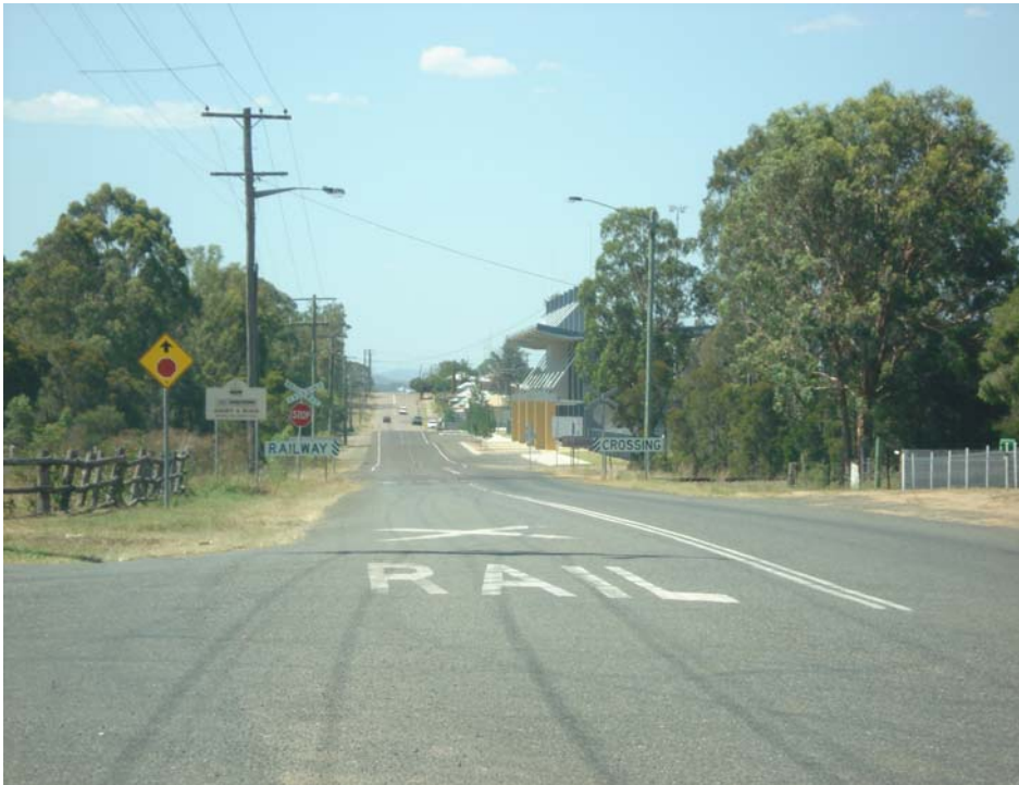
Photo 1-2 Southern Approach to Level Crossing
