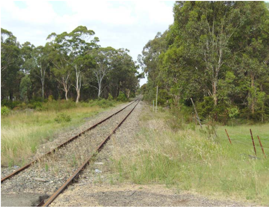
Photo 1-4 View to The East Along Rail Line From Level Crossing
