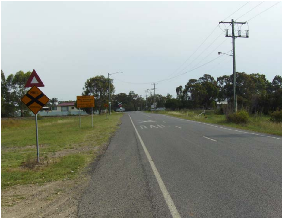
Photo 1-1 Northern Approach to Level Crossing
