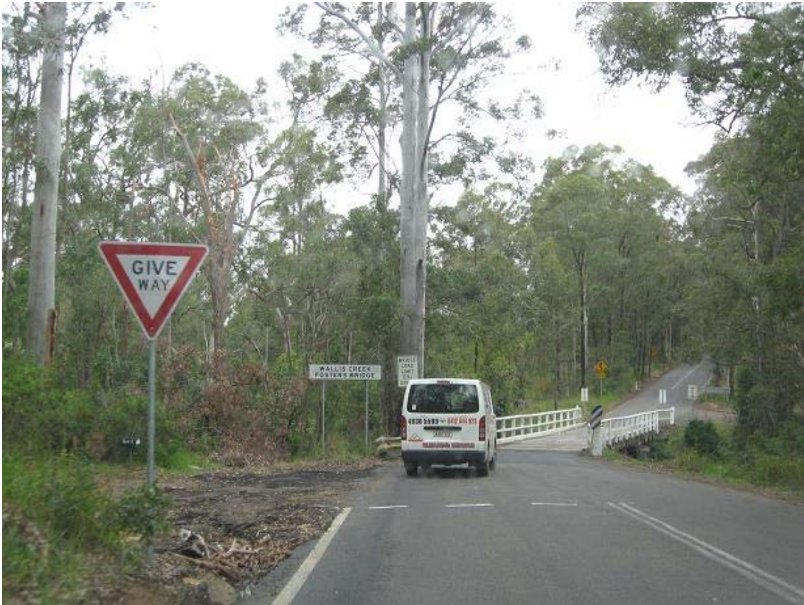
Photo 2 Wallis Creek Fosters Bridge – Sandy Creek Road
