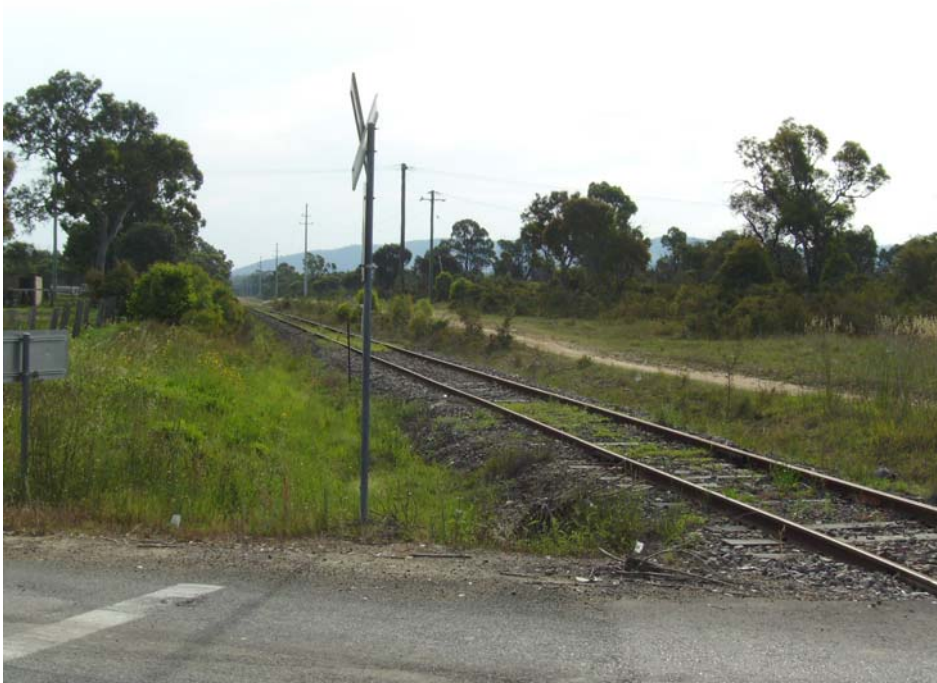
Photo 1-3 View to The West Along Rail Line From Level Crossing
