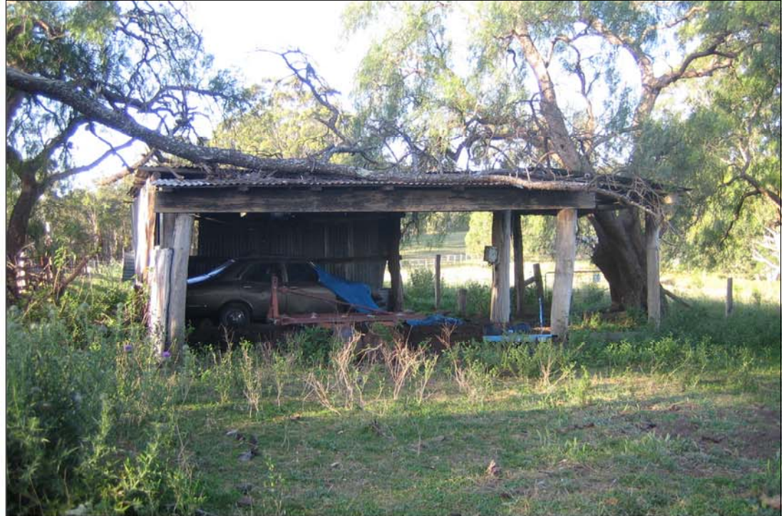
PLATE 16 View showing garage/shed at former house site (Item 15)
