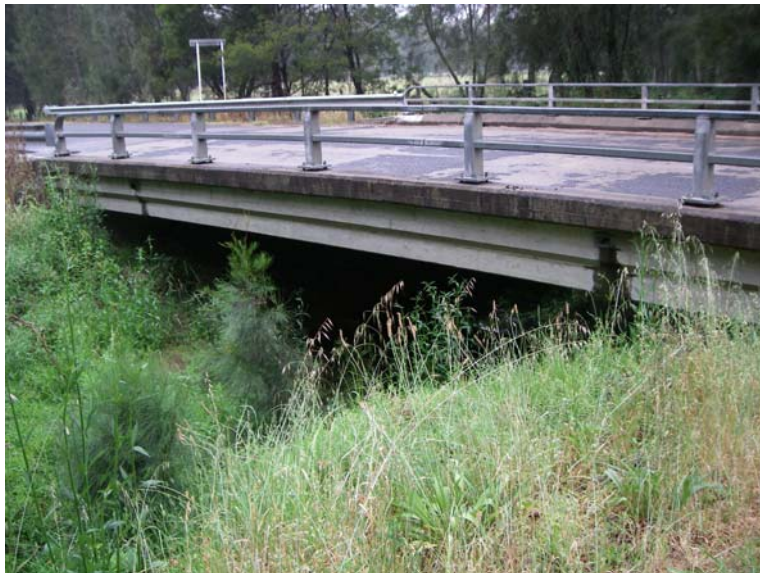
Fig. 6.4 Bridge BR-SR01 along Sandy Creek Road
