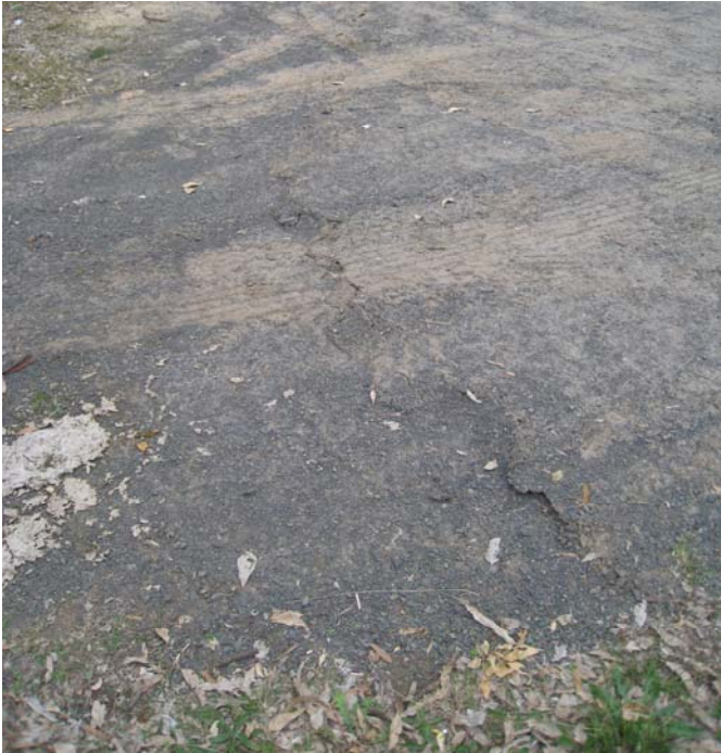
Fig. 4.12 Example of Surface Compression Buckling Observed in Road Pavement (Observed in the Southern Coalfield at a Similar Depth of Cover as the Study Area)
