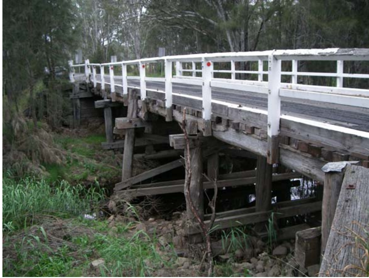
Fig. 6.3 Bridge BR-QR01 along Quorrobolong Road
