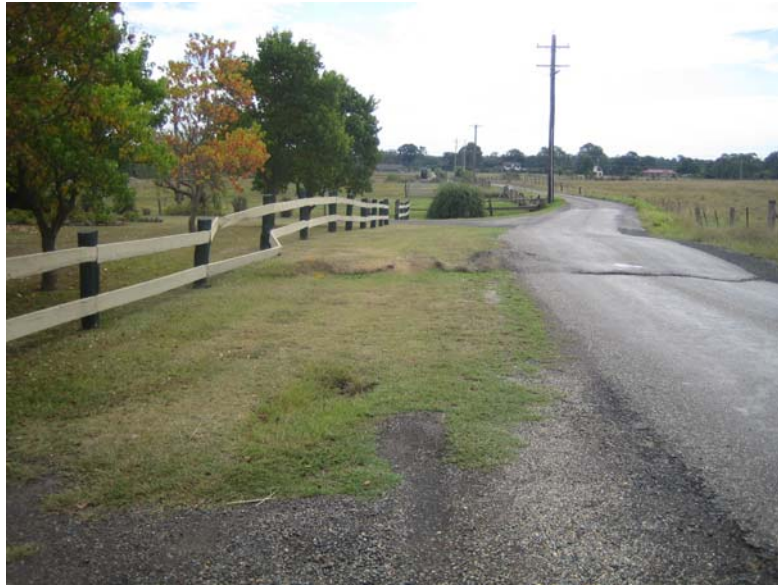
Fig. 5.8 Example of Surface Compression Humping due to Low Angle Thrust Fault
