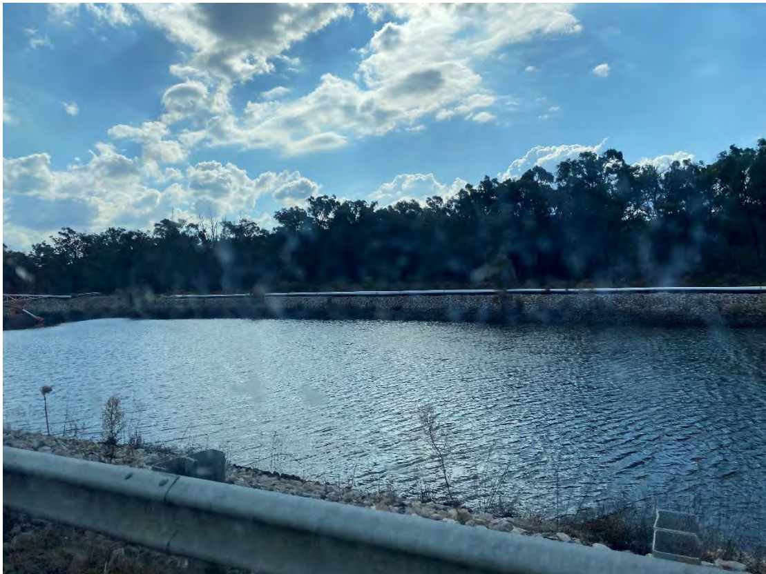
Plate 16 – Sediment dam from Open Cut 1 stockpile
