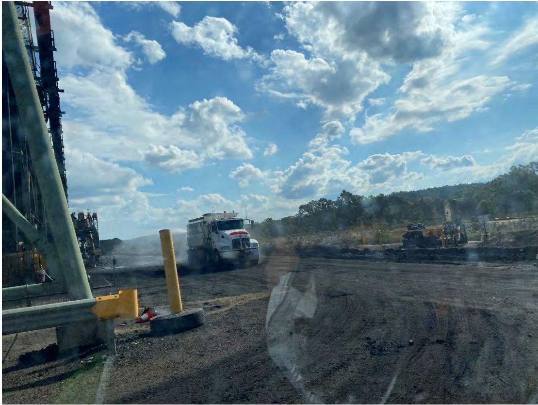
Plate 15 – Water cart in operation outside CHPP
