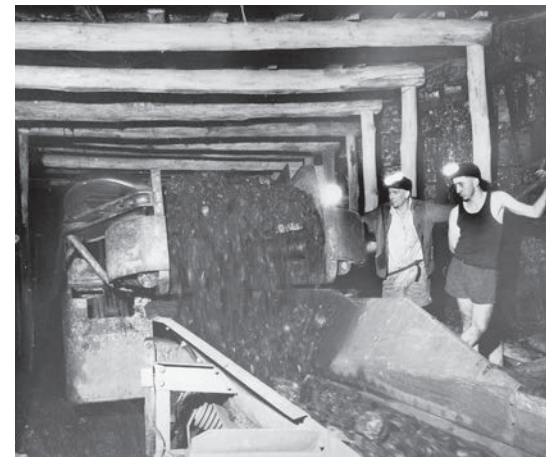
UNLOADING A SHUTTLE CAR OF COAL AT THE CONVEYOR BOOT END, NOVEMBER 1957. PHOTO: M. BARRETT COLLECTION
