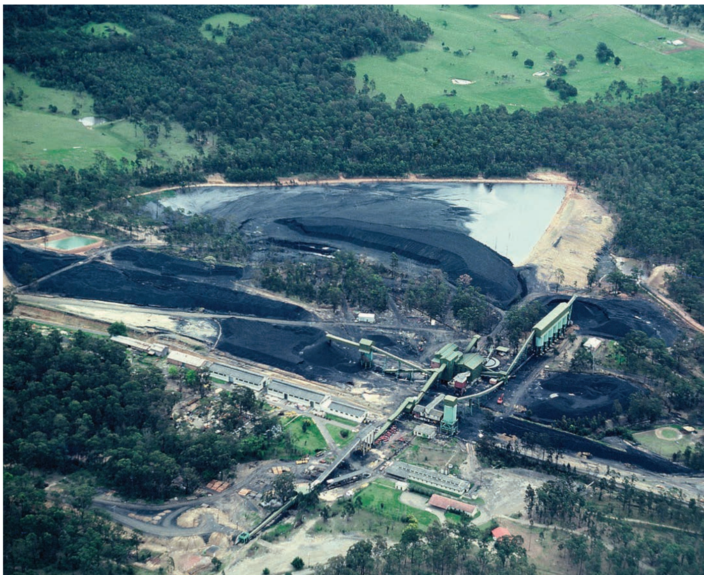
ELLALONG COLLIERY'S OVERLAND CONVEYOR PRIOR TO THE INSTALLATION OF COVER, CIRCA 1979. PHOTO: NEWCASTLE WALLSEND COAL COMPANY
