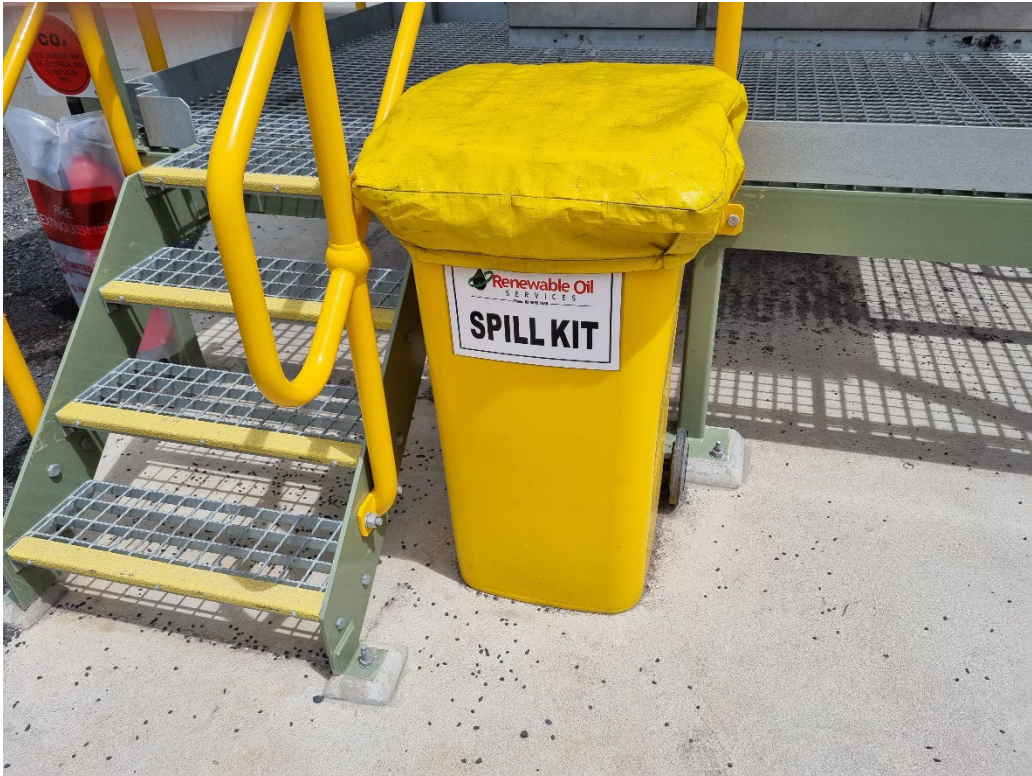
Photograph 18 - Spill Kit (at bulk fuel storage bund)
