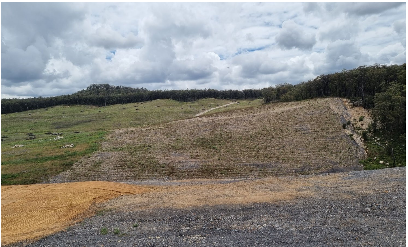
Photograph 10 - Progressive Rehabilitation Works at OC4
