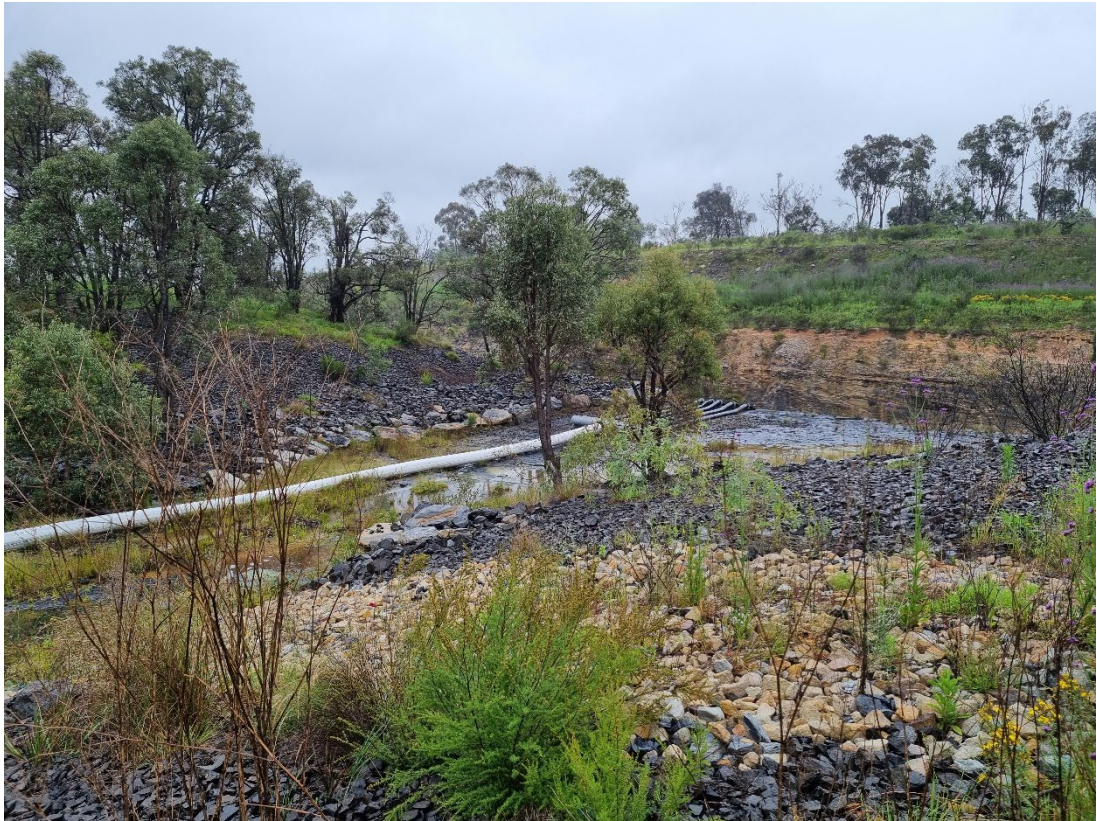
Photograph 12 - Water Treatment Plant Discharge to Goulburn River
