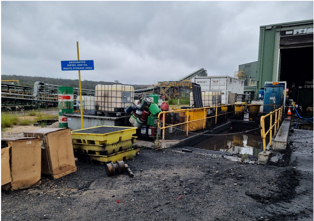
Photograph 9 - Waste Oil Storage Area at Coal Processing Plant
