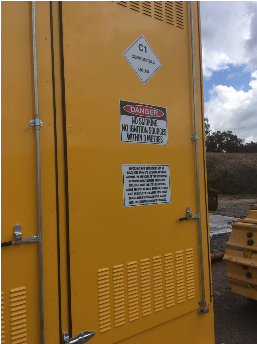
Combustible liquid storage
