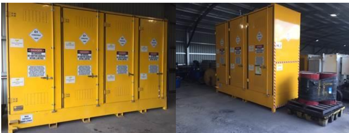
Combustible liquid storage
