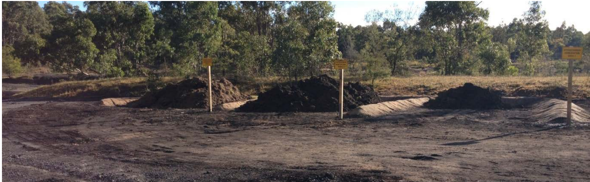
FIGURE 2.1 HYDROCARBON REMEDIATION AREA
