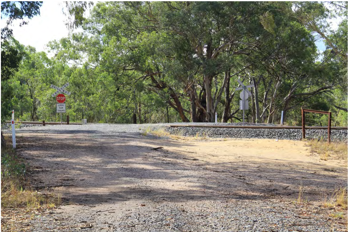
Photograph B-9: LXM 1298 Northbound along Local Road
