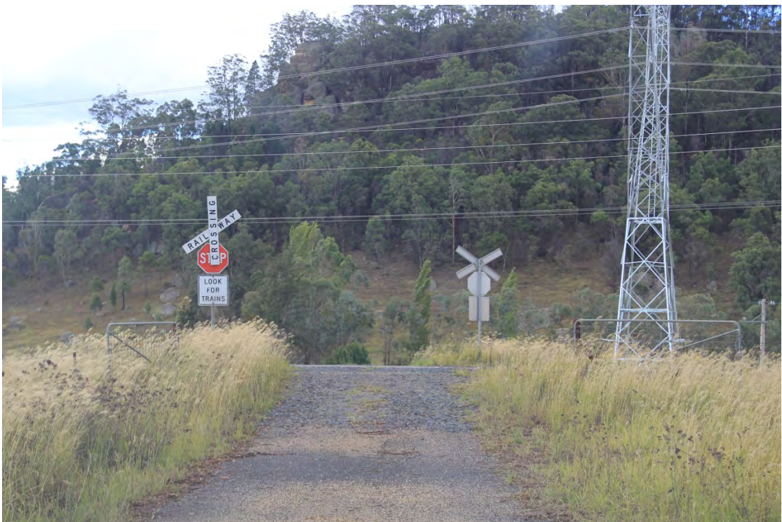
Photograph B-3: LXM 1302 Northbound along Local Road
