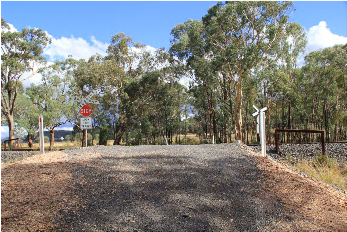
Photograph B-10: LXM 1298 Southbound along Local Road
