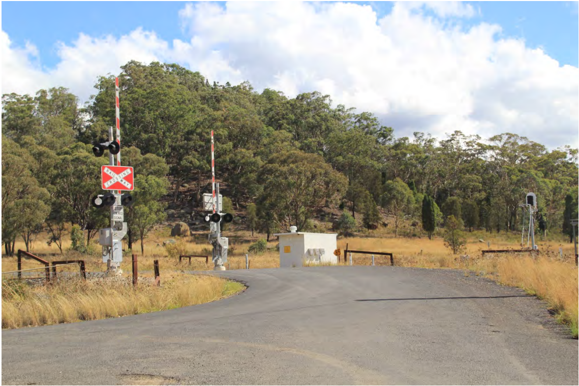
Photograph B-12: LXM 1297 Southbound along Mogo Road
