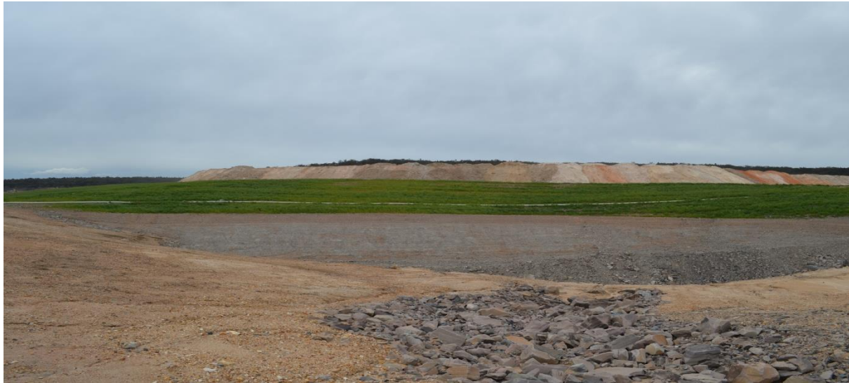
Figure 65: Rehabilitation Trial Location and Set Up
