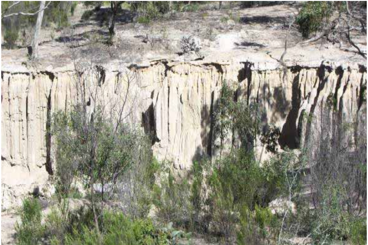
Plate 3 VIEW LOOKING EAST FROM ULAN ROAD SHOWING SEVERE EROSION ALONG THE UPPER REACHES OF RYANS CREEK
