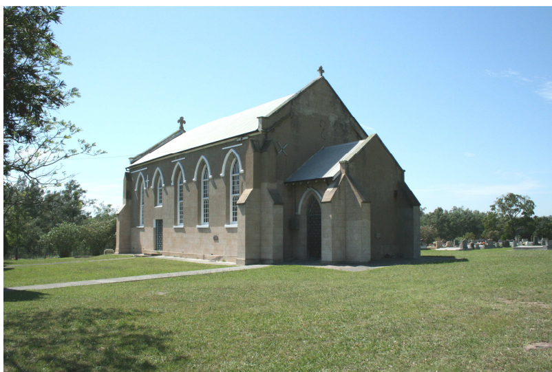
Photograph 1 St Clement's Anglican Church source: Heritas 2008
