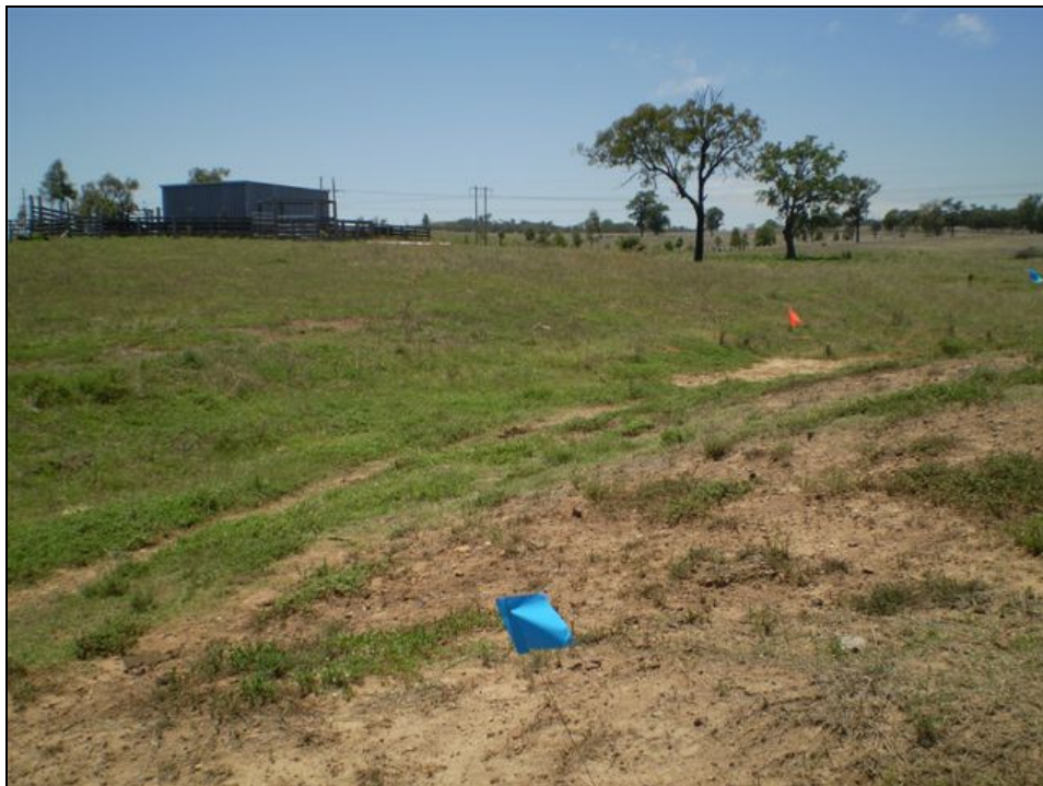
Plate 12 - View north across dam in SA9
