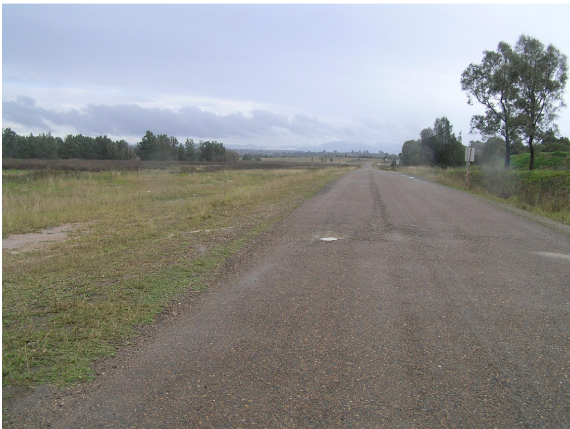
Figure 16: Sealed section of Brunkers Lane.
