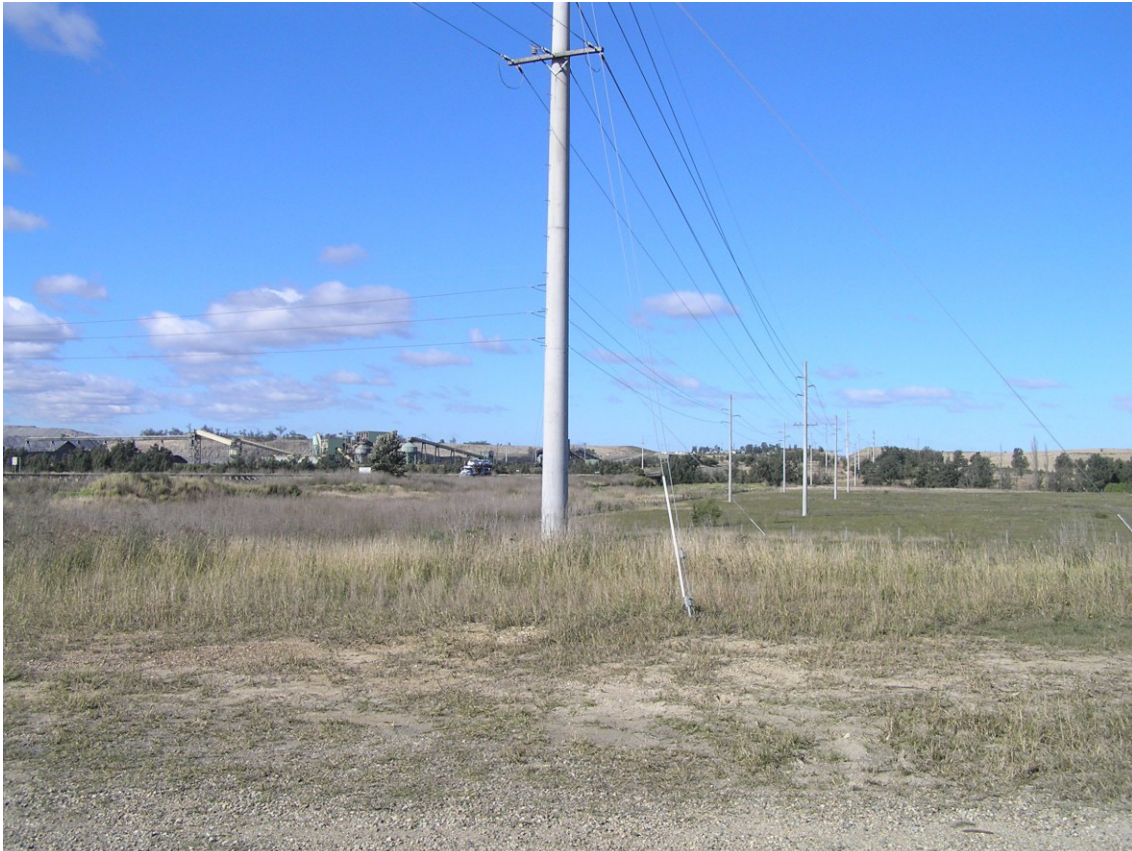
Figure 10: Photograph looking east along New England Highway road reserve.
