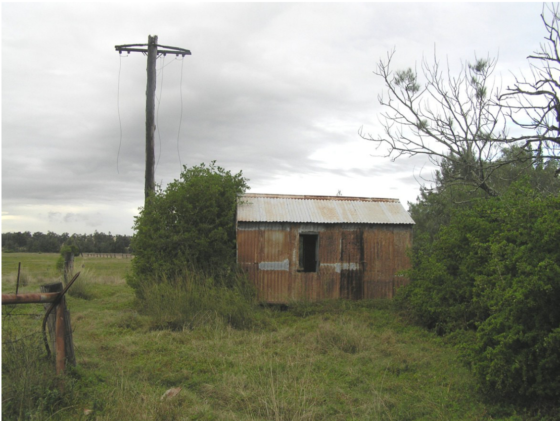
Figure 22: Disused pump shed adjacent to Bowmans Creek.
