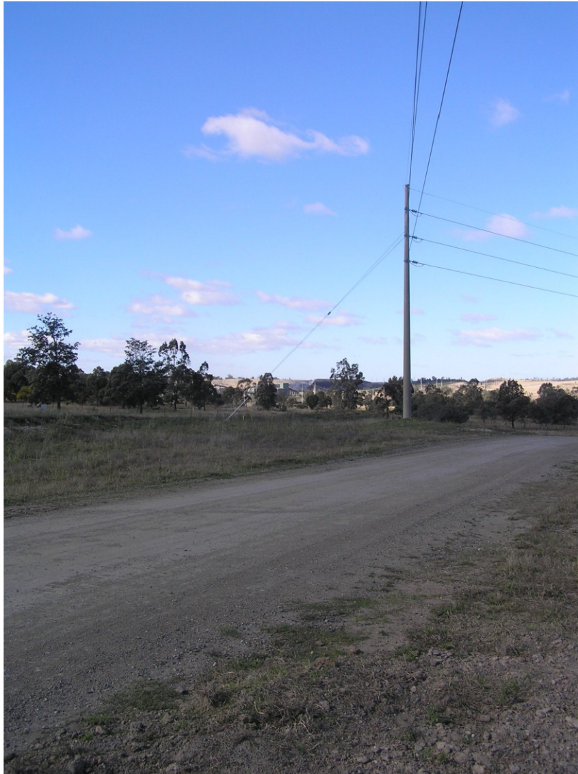
Figure 17: Unsealed access road on Macquarie Generation lease.
