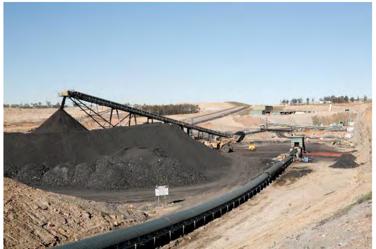
Underground RC conveyor and ROM
