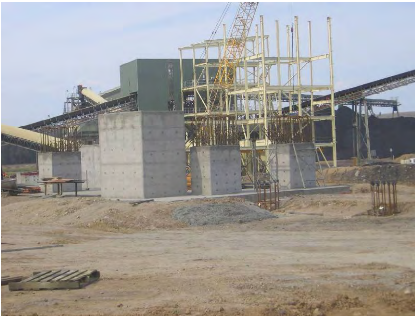
Module 2 Breaker Station Foundations
