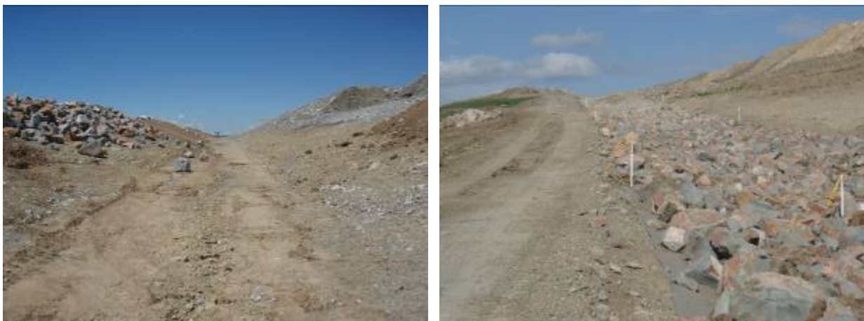
Figure 5. Northern drop structure under construction
