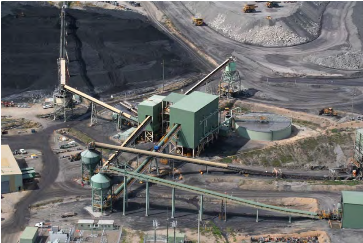
Figure 3. Coal Handling Preparation Plant
