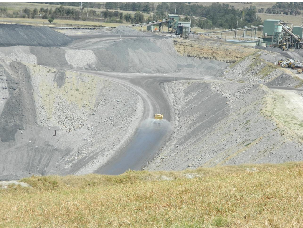
Photograph 8 – Water cart operating on haul road into former NEOC pit
