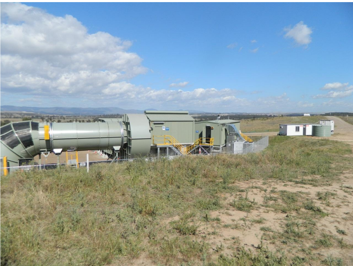
Photograph 2 – Upcast Ventilation Shaft site
