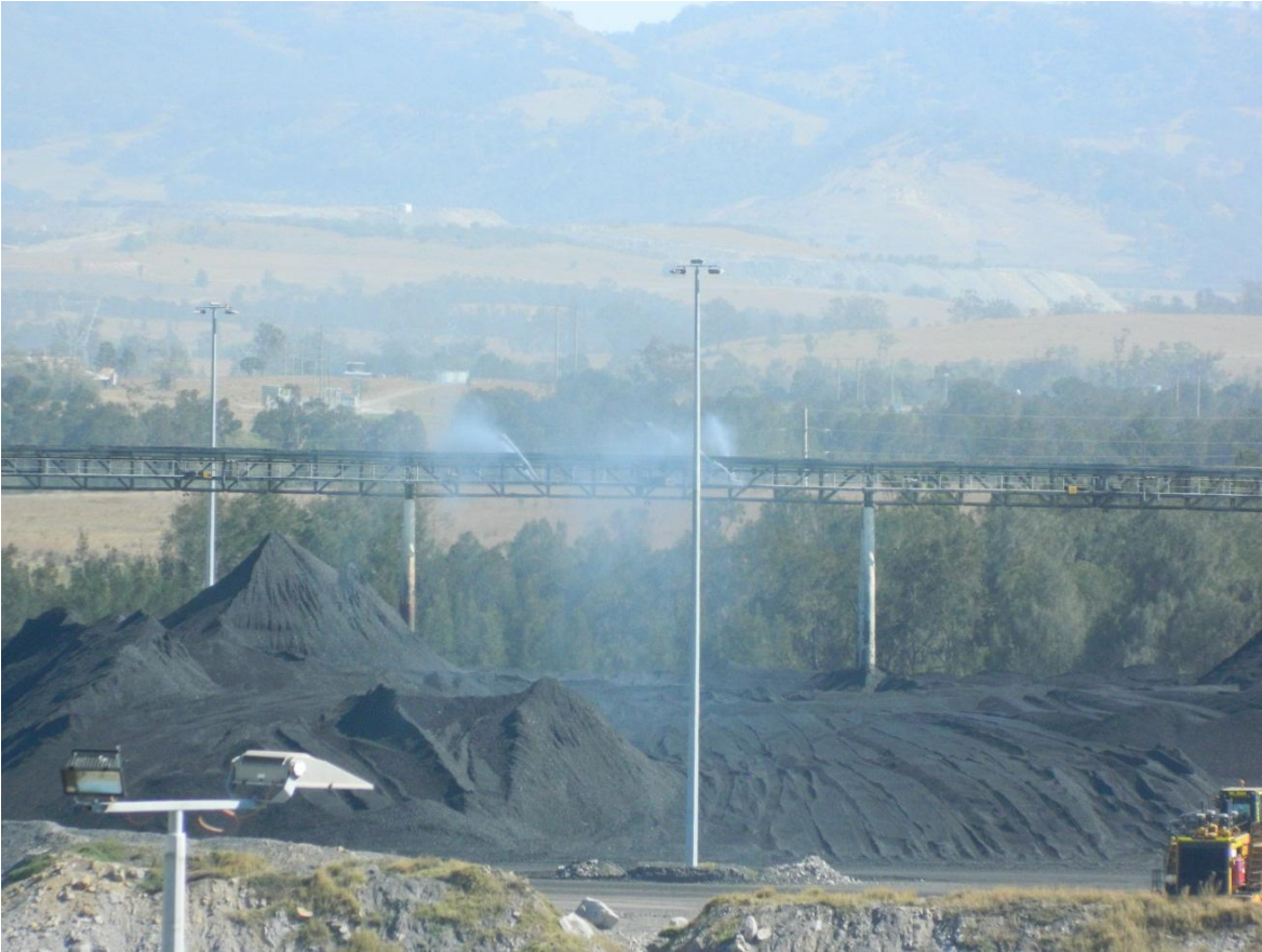
Photograph 9 – Automatically activated sprays over product coal stockpile
