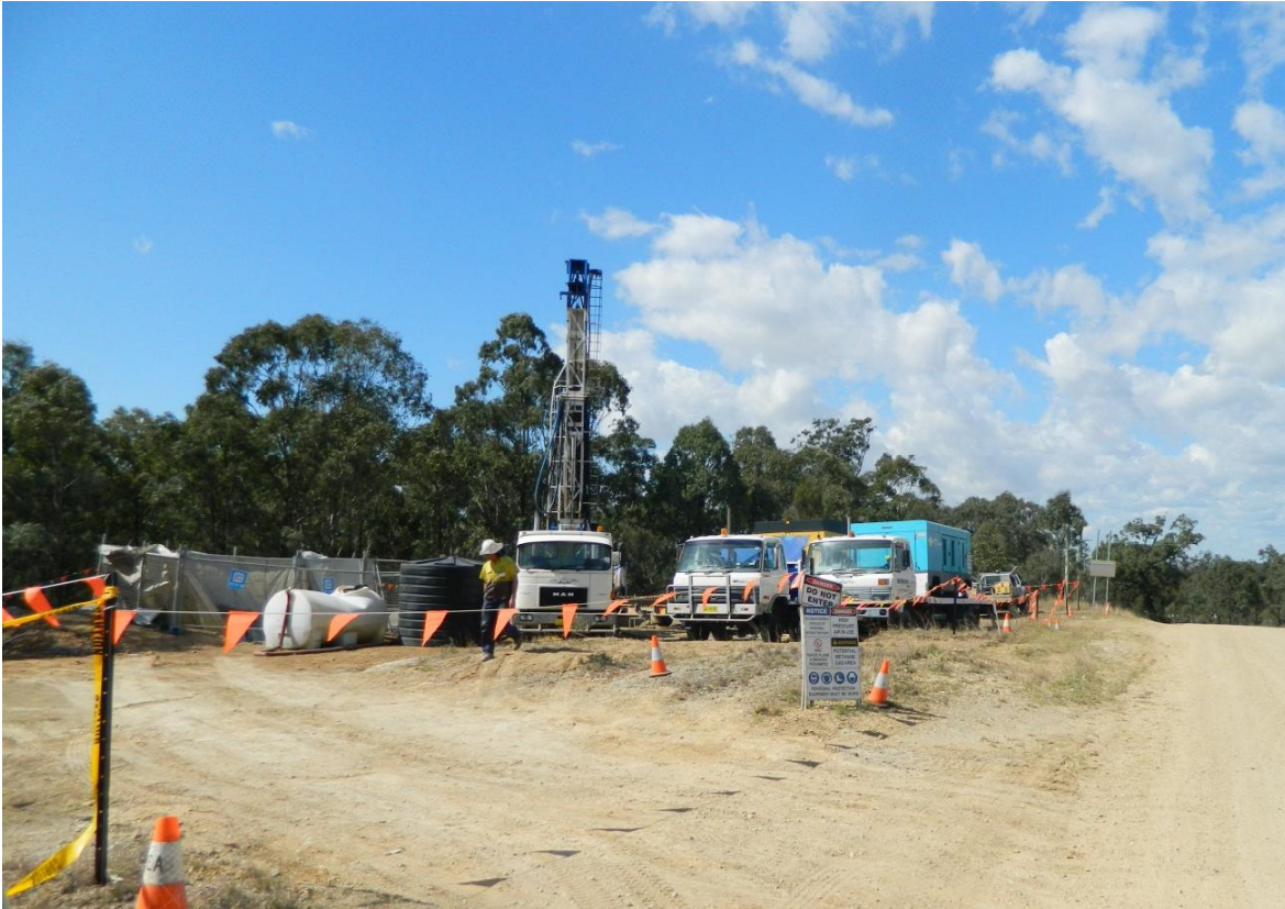
Photograph 3 – Large diameter gas drainage drill site on Dairy Lane
