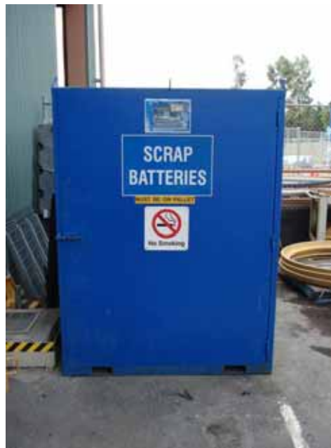
Used batteries are stored inside DG rated Battery storage unit on pallets
