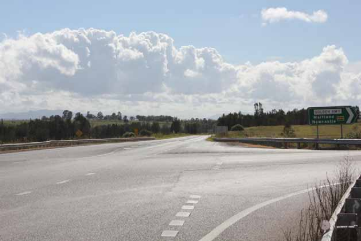
Photograph 2.1 Golden Highway/Mitchell Line Road intersection looking east
