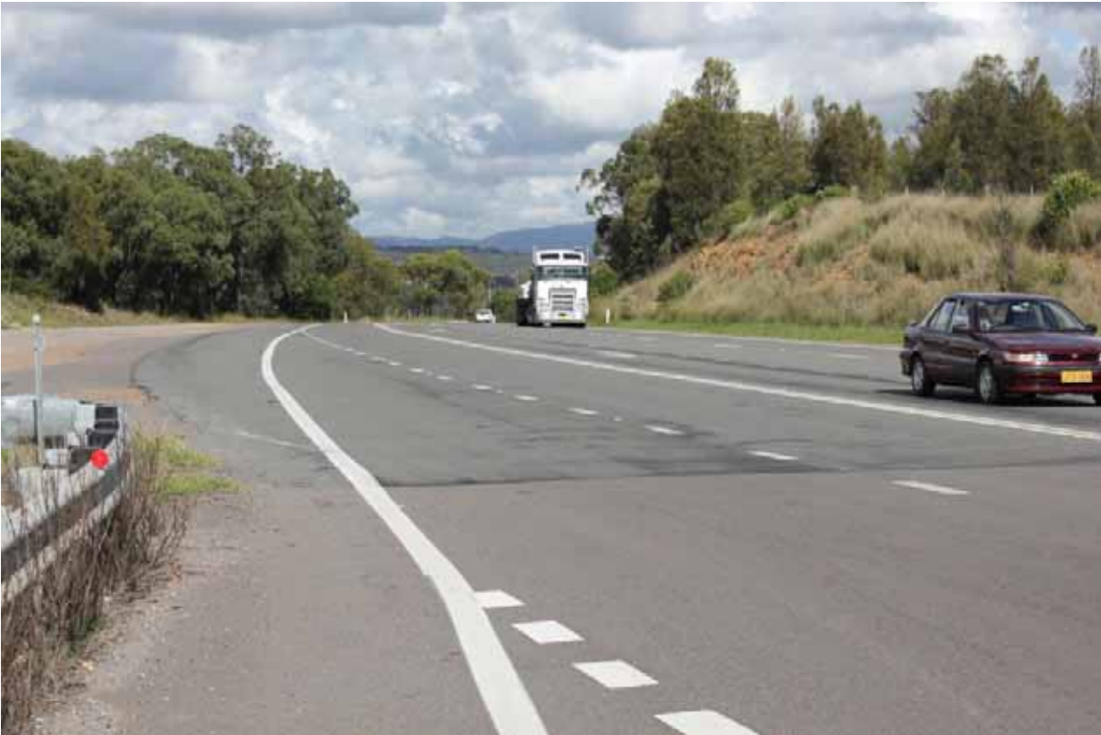
Photograph 2.2 Golden Highway/Mitchell Line Road intersection looking west
