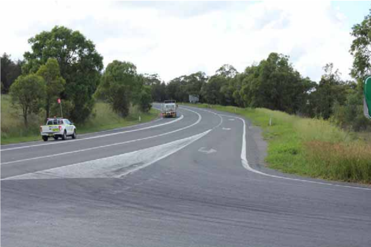
Photograph 2.3 Golden Highway/Broke Road intersection looking east
