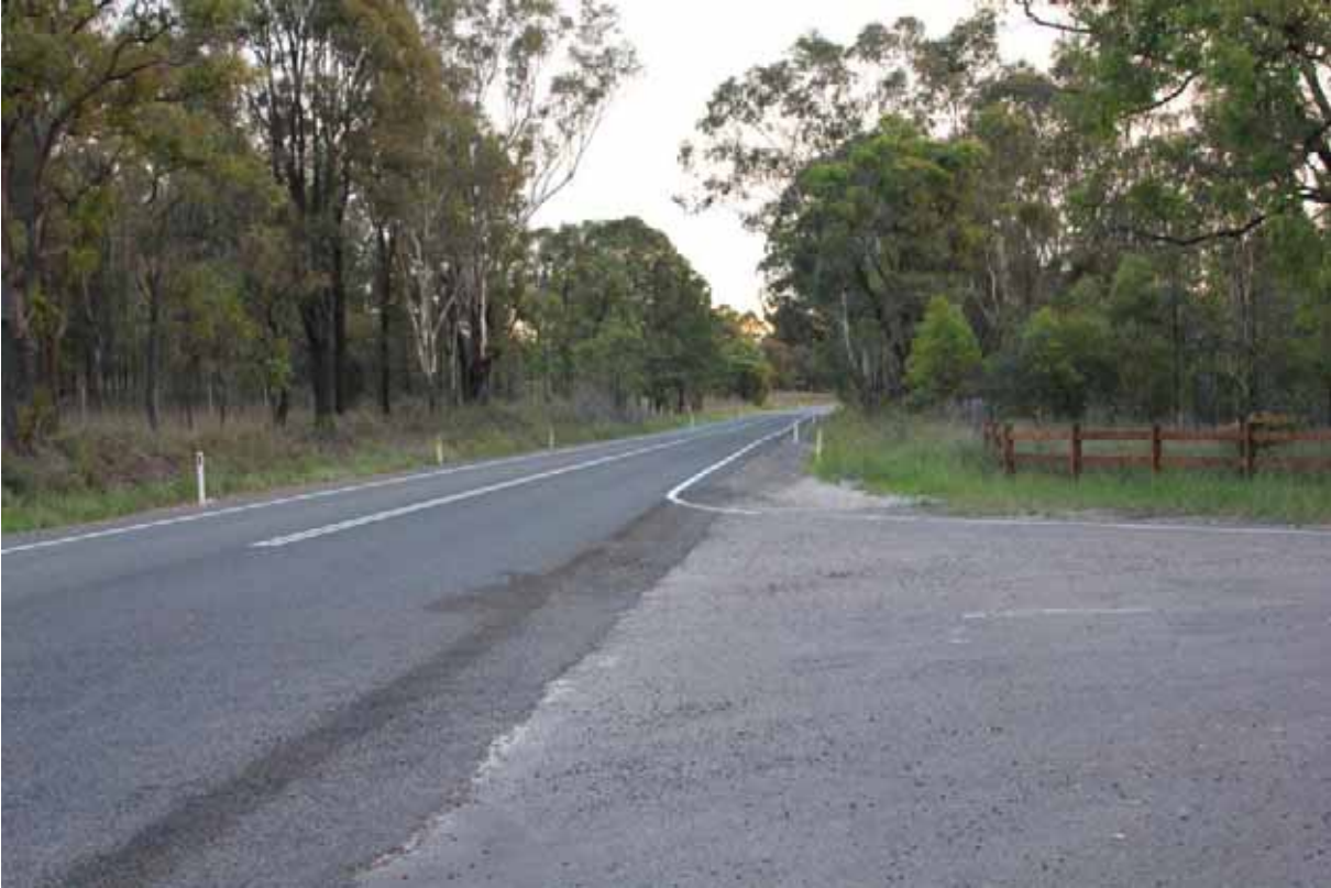
Photograph 2.7 Broke Road/MTO CHPP access intersection looking south
