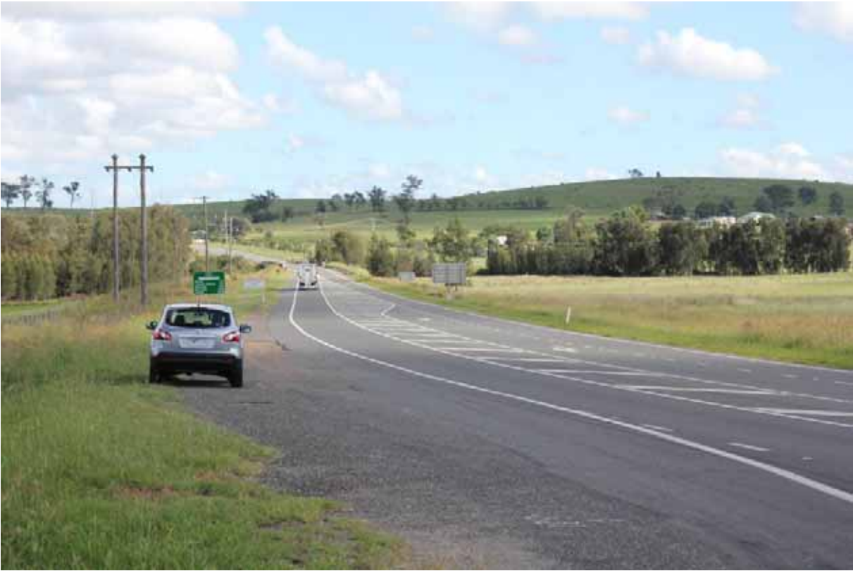
Photograph 2.4 Golden Highway/Broke Road intersection looking west
