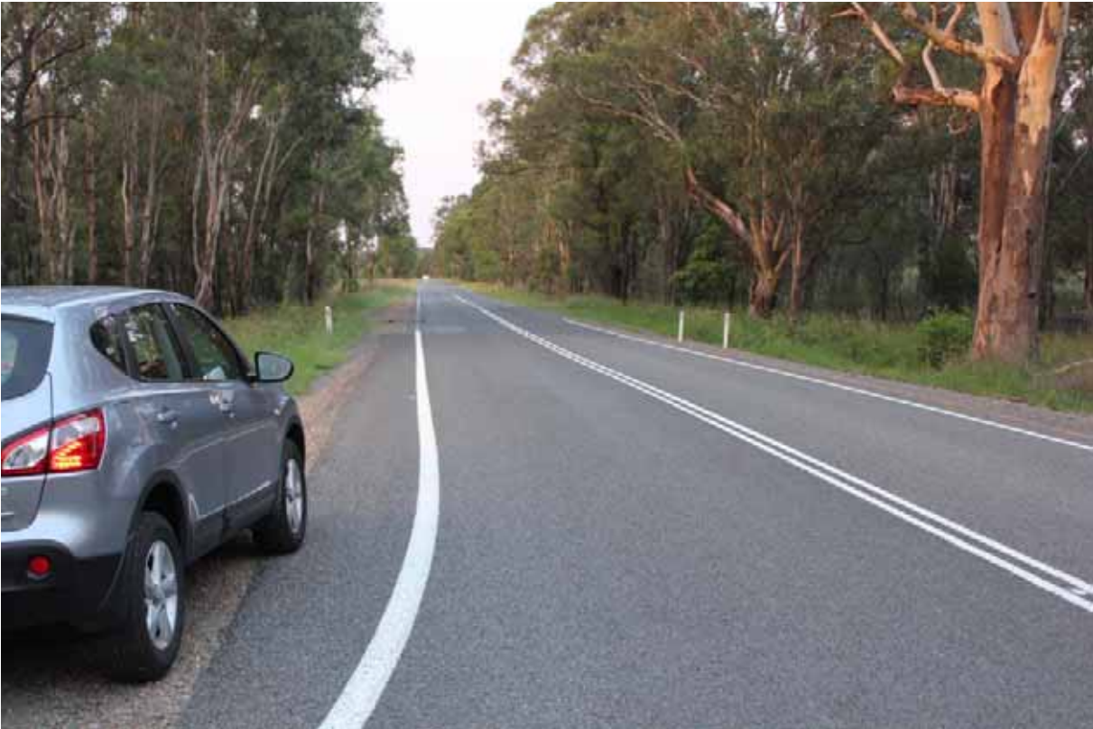
Photograph 2.8 Broke Road/MTO CHPP access intersection looking north
