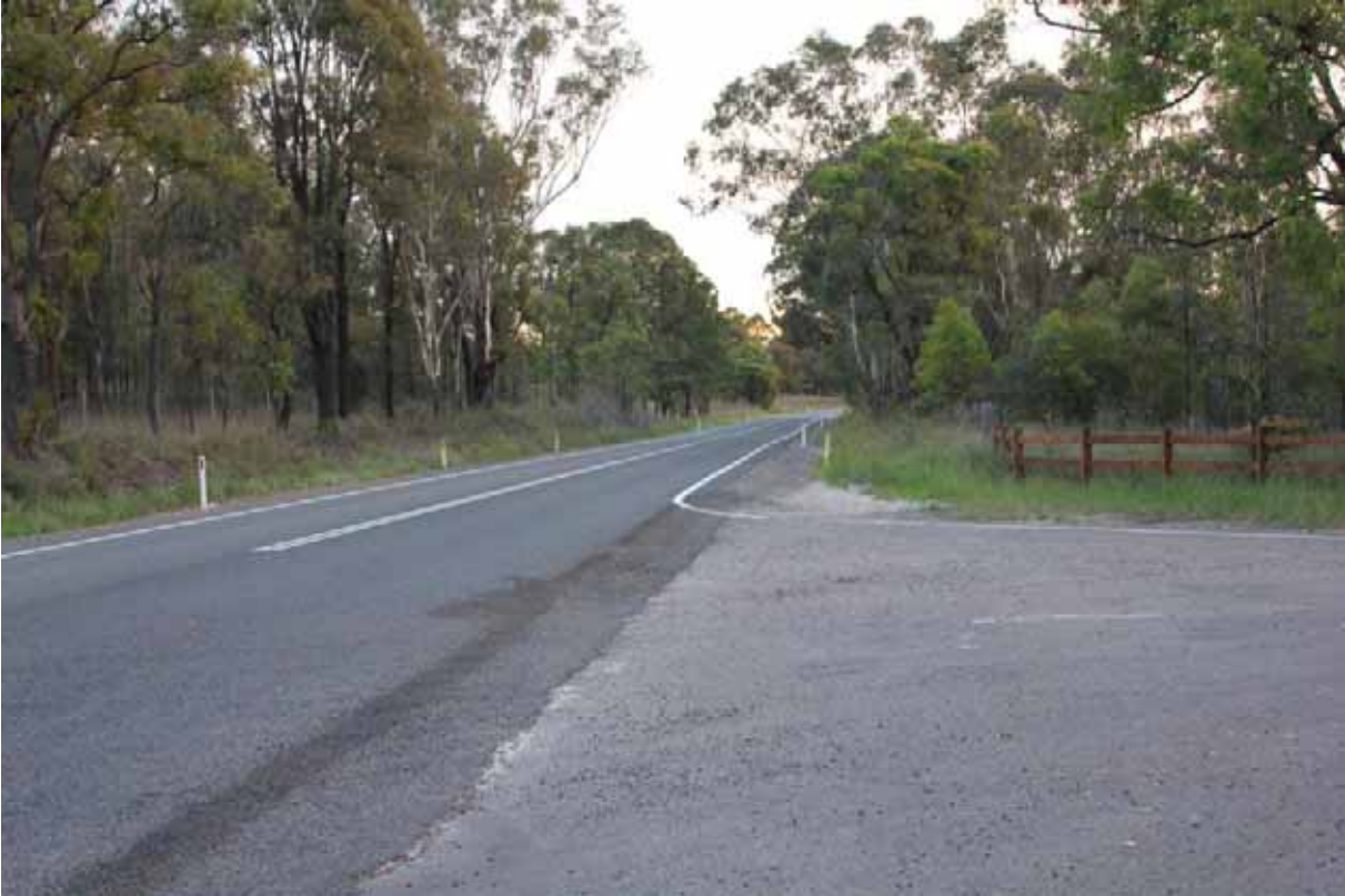
Photograph 2.7 Broke Road/MTO CHPP access intersection looking south
