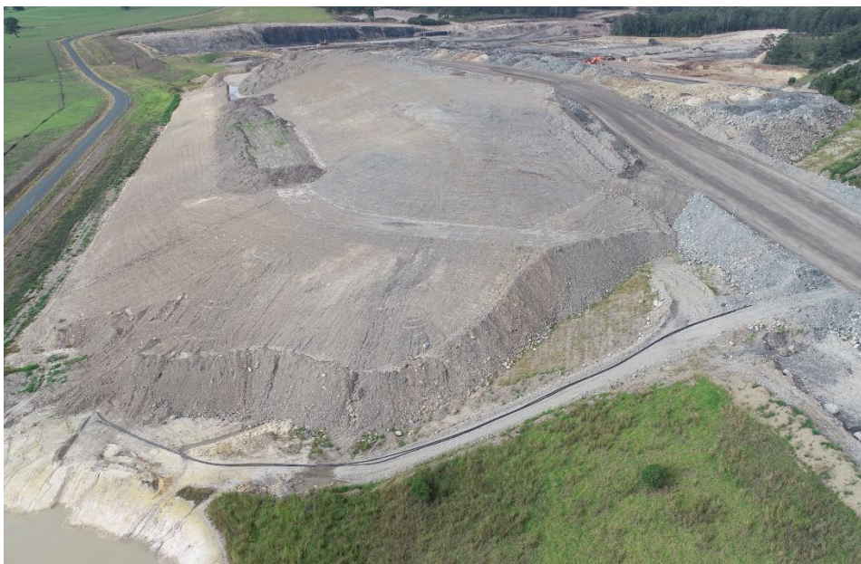
Photo: Bulk shaping on the Avon North Waste Emplacement, May 2019.
