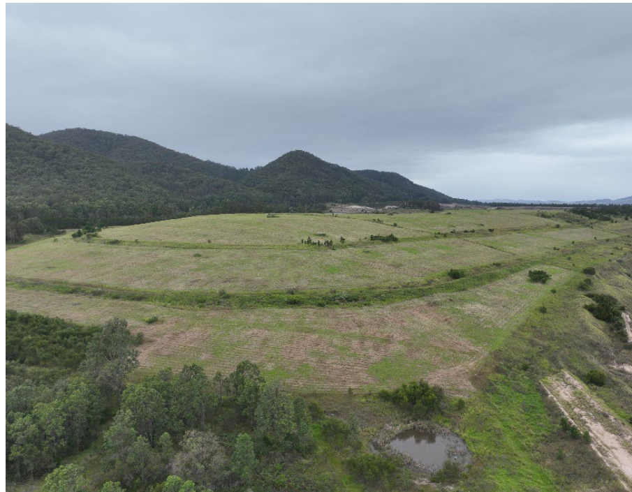
Plate 1: OMP Rehabilitation Maintenance. March 2024.
