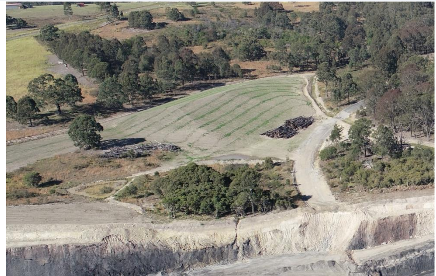
Photo: Avon North clean water diversion drain and backfilled area, July 2019.
