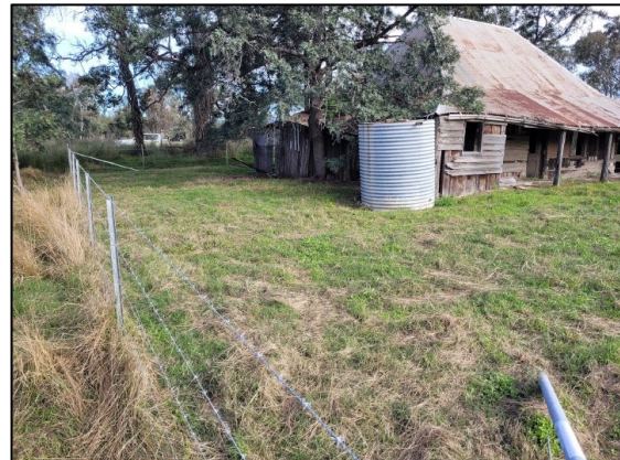
Springwood homestead following grounds maintenance
