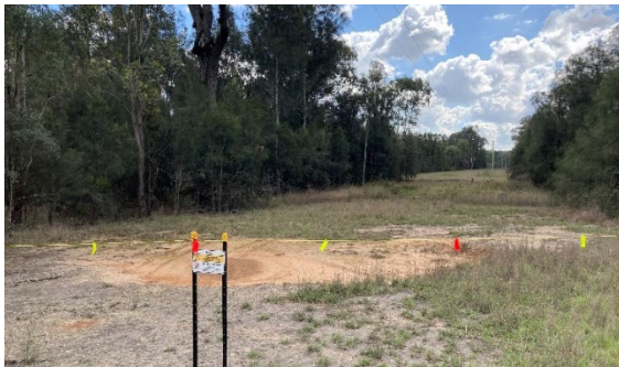
Example of barricading and signage being replaced
