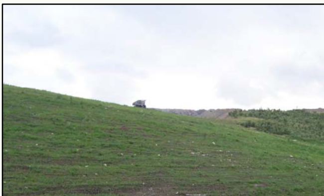
C Duralie Coal Mine Waste Rock Emplacement Revegetation Looking North
