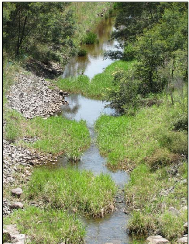
Coal Shaft Creek Diversion Looking Upstream from Haul Road Culvert
