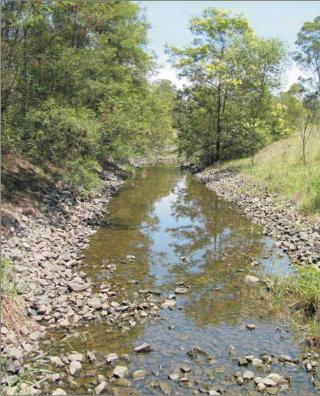
Coal Shaft Creek Diversion Looking Upstream
