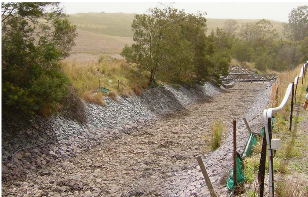
Plate A-2 – Typical Rockfill Mattress-Lined Channel Shortly After Construction
