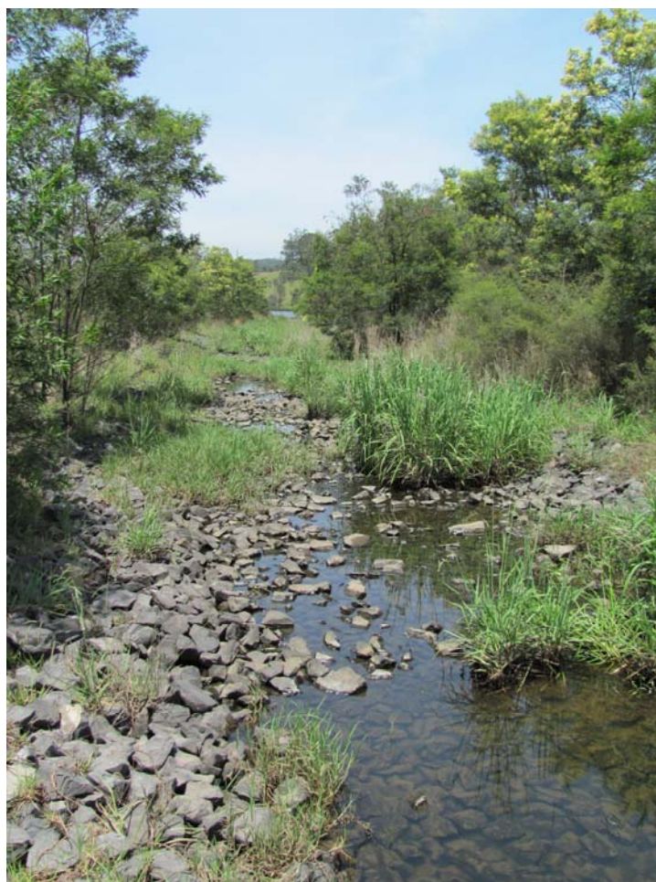
Plate A-4 –Diversion Channel Looking Downstream to Dam 1 (November 2009)
