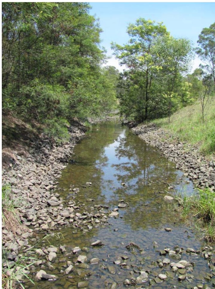
Plate A-5 –Diversion Channel Looking Upstream to Dam 3 (November 2009)
