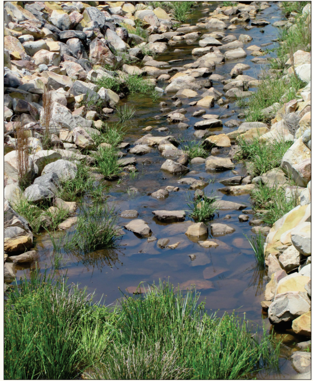
Coal Shaft Creek Diversion Looking Downstream
