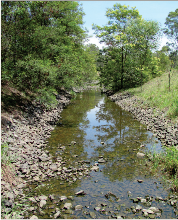
Coal Shaft Creek Diversion Looking Upstream
