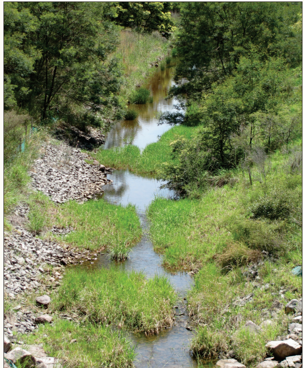
Coal Shaft Creek Diversion Looking Upstream from Haul Road Culvert
