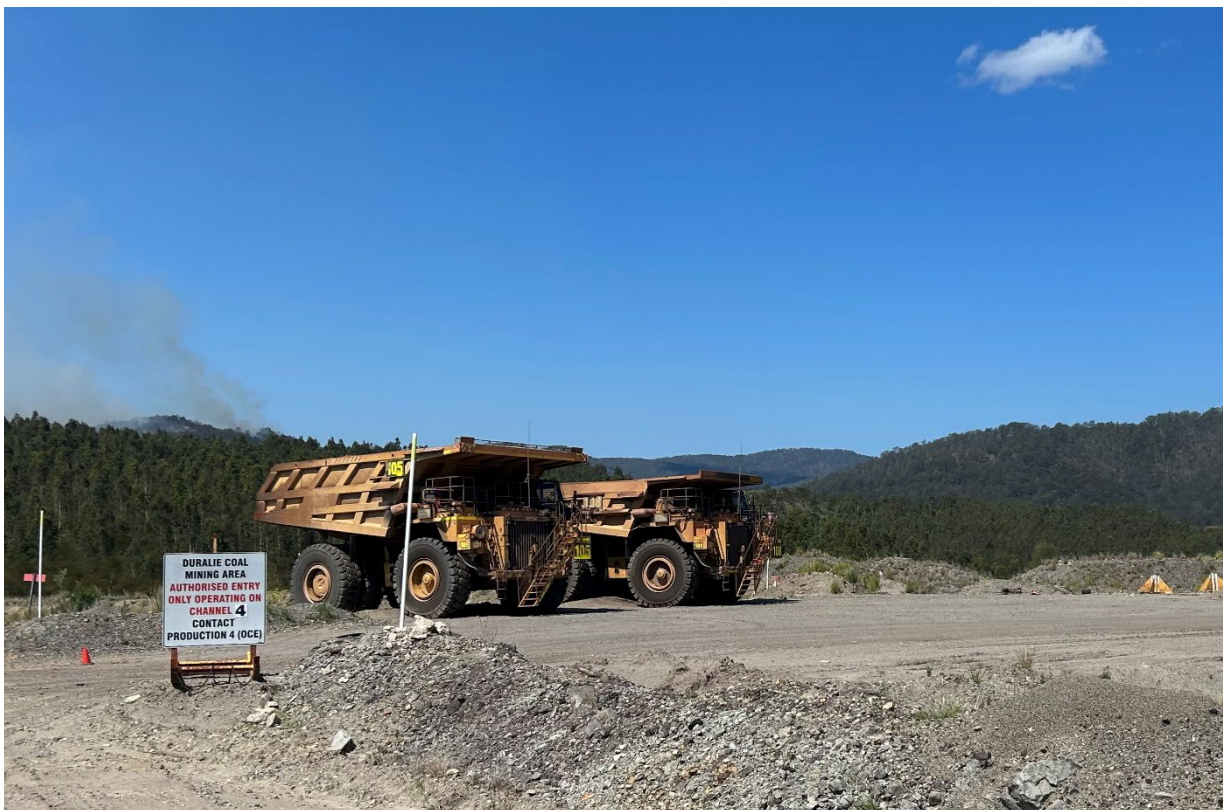
Plate 8 – Dump trucks remaining on site for potential use in rehabilitation (bushfire in background)
