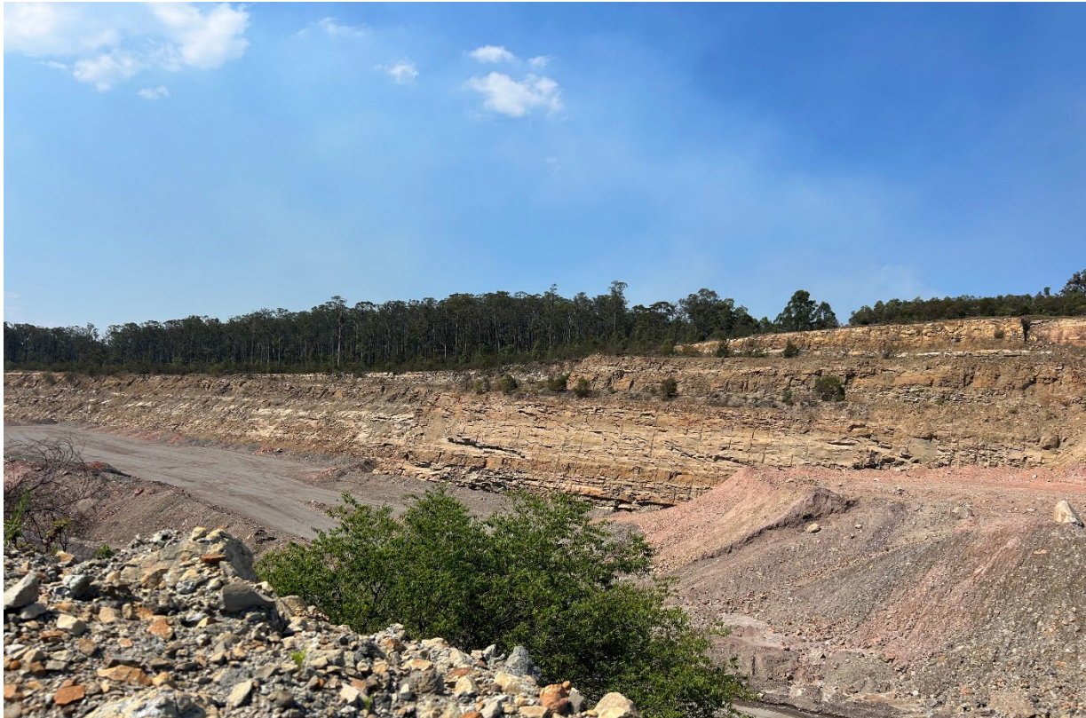
Plate 9 – PAF pumping area in Weismantel pit
