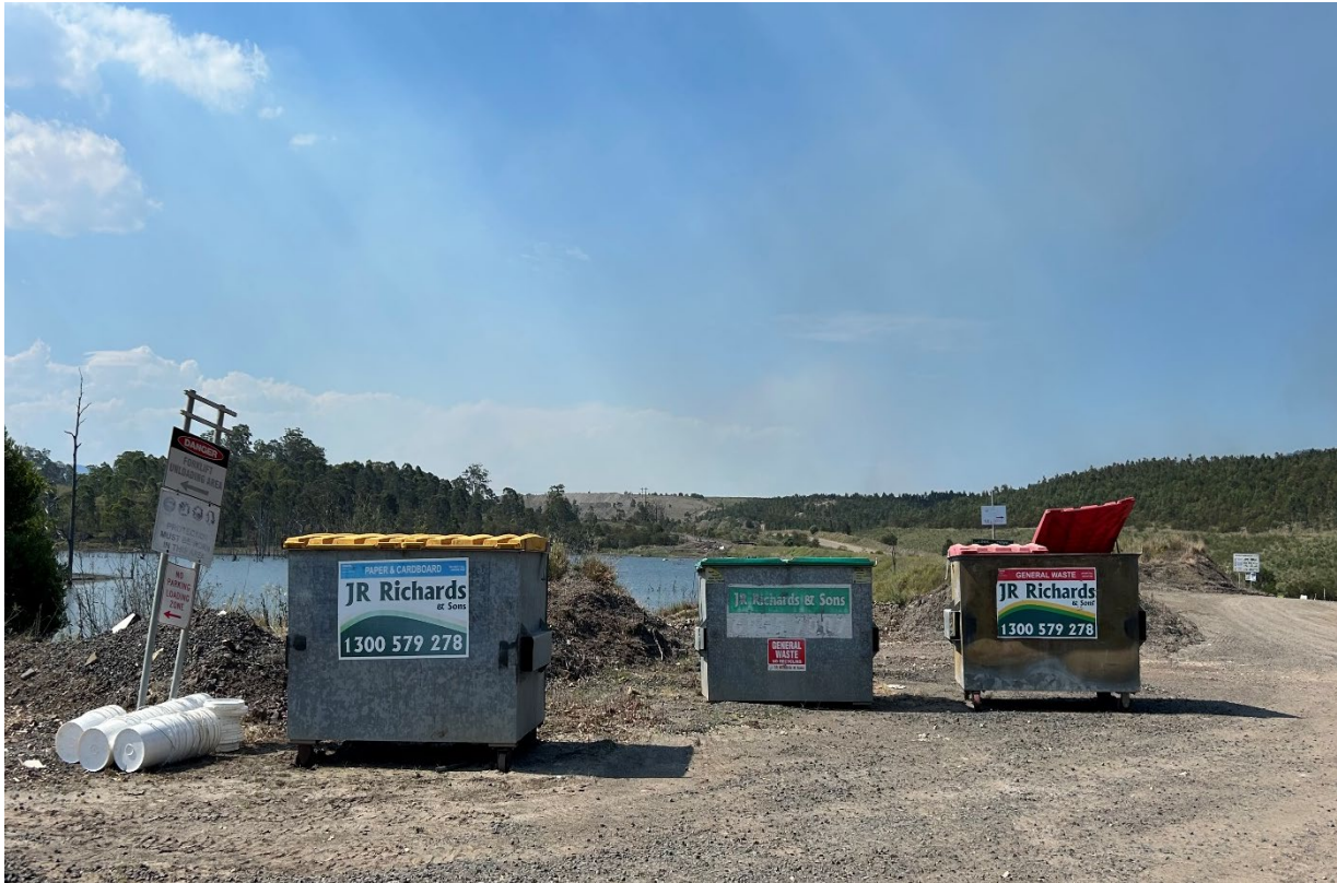
Plate 13 – Segregated waste bins near site office
