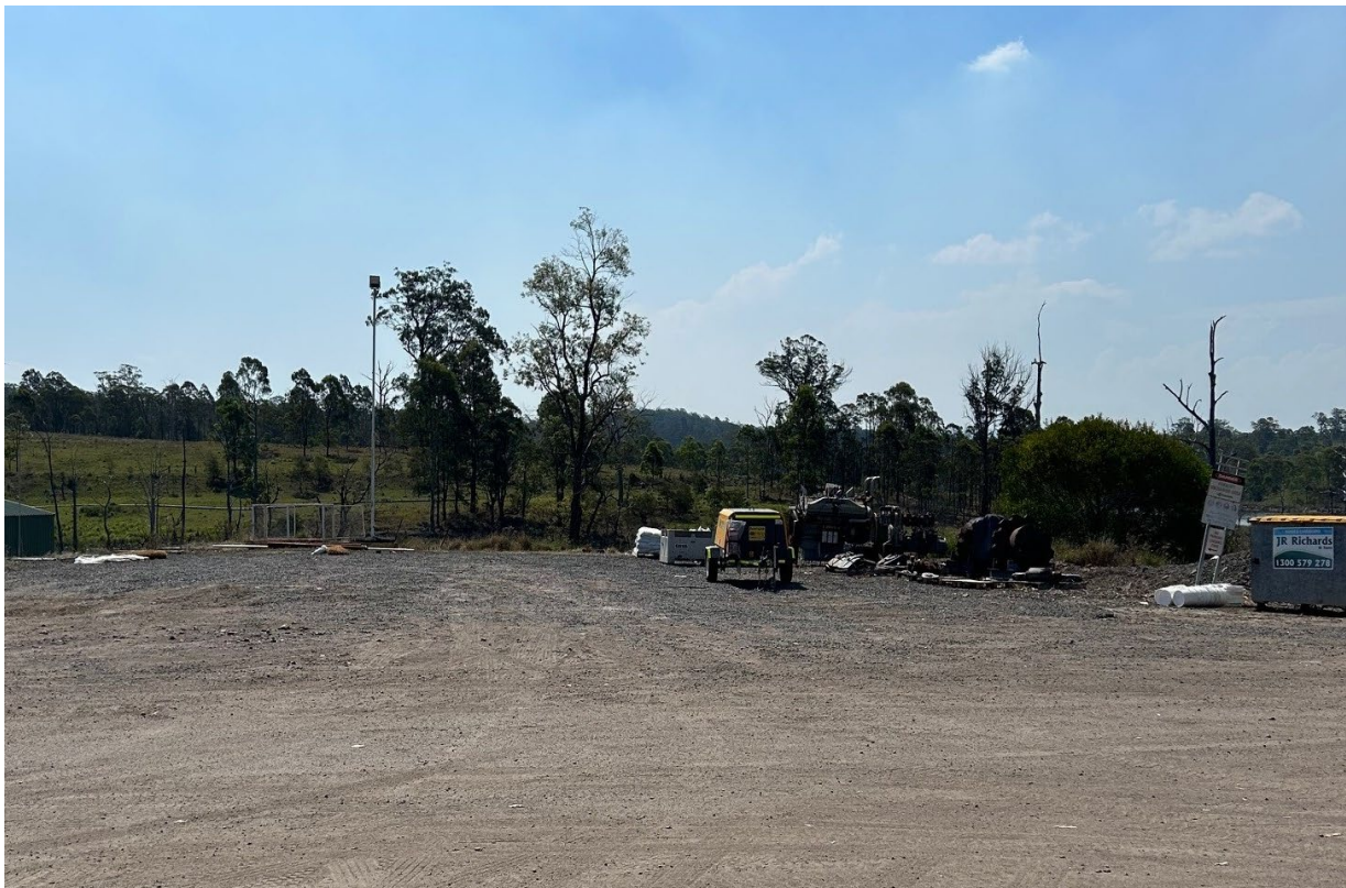
Plate 18 – Minimal waste stored near site office requires minimal housekeeping
