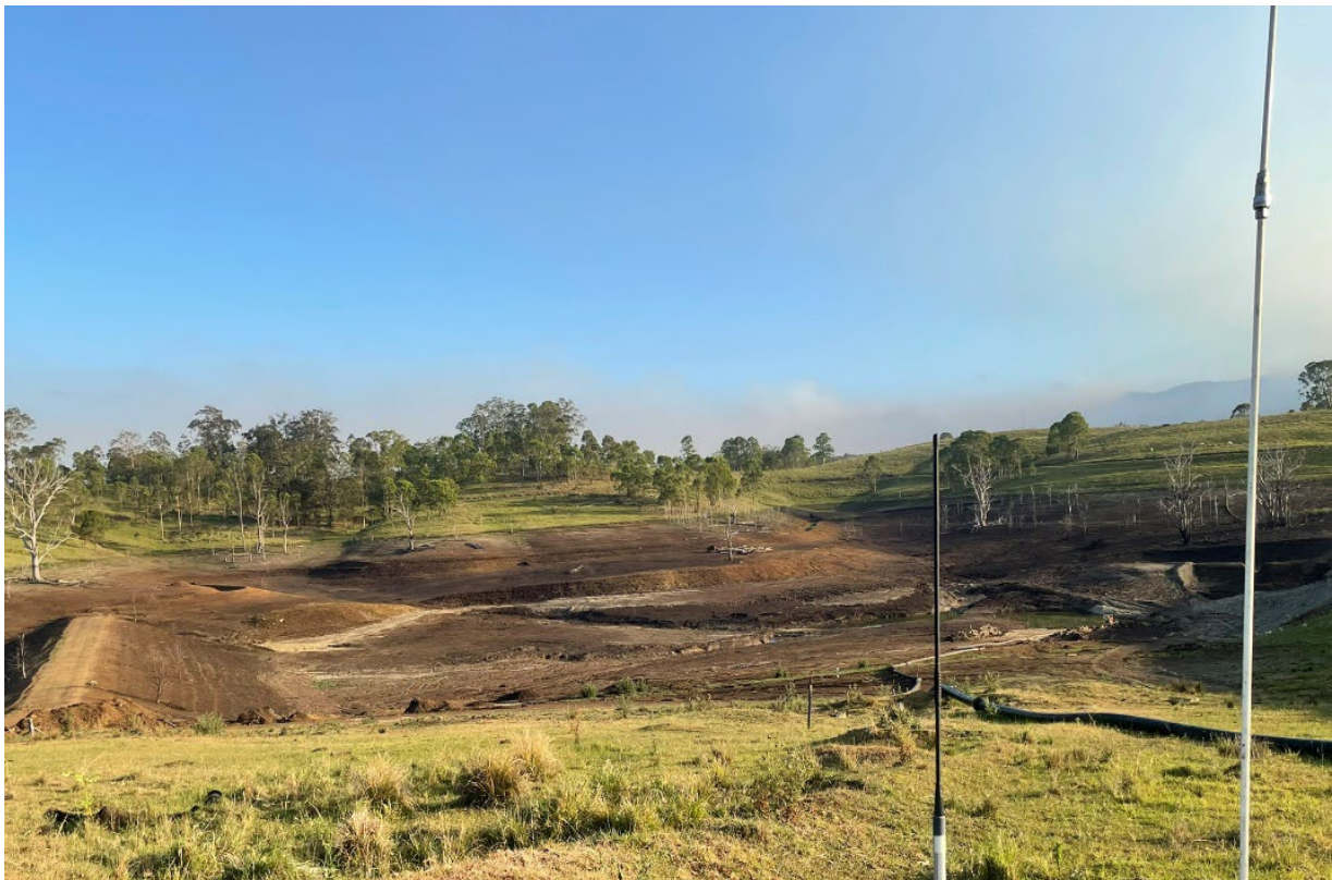
Plate 4 – Auxiliary Dam 2 undergoing decommissioning (Minesoils, 2023)
