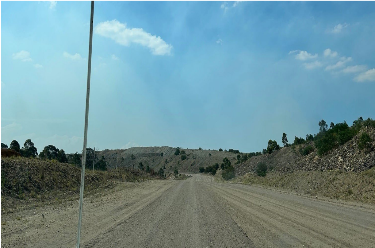
Plate 15 – Haul road view with temporary vegetation
