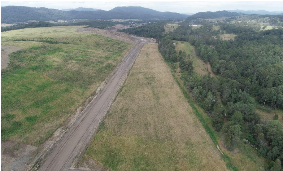
Photo: Complete rehabilitation at Weismantel waste emplacement and Duralie Haul Rd, taken May 2021.
