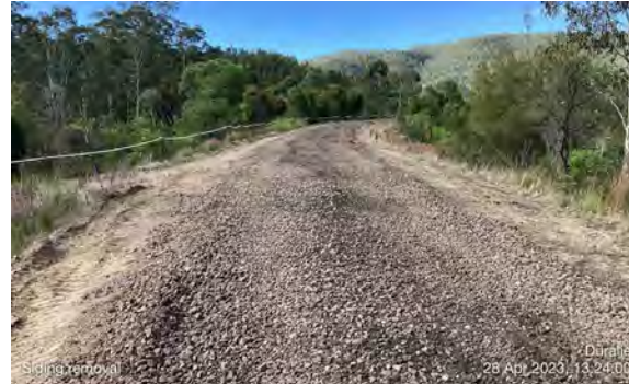
Duralie Rail and Sleepers removed
