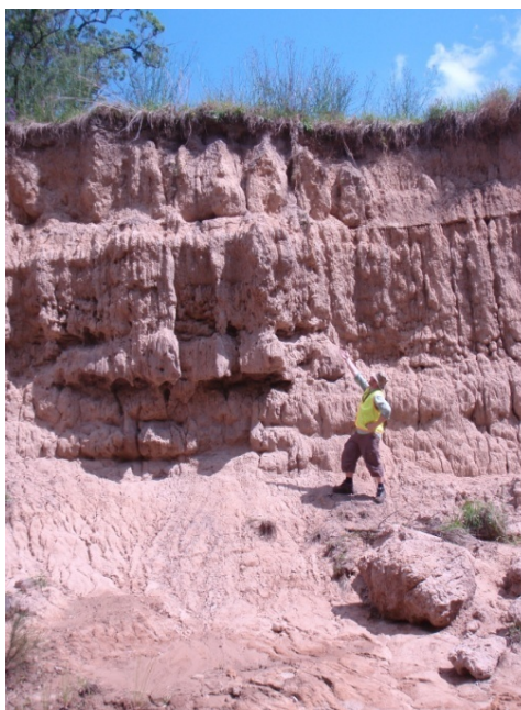
Plate 2: Bank erosion in Vegetation Management Unit A
