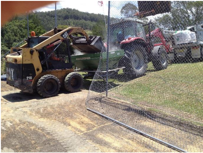
Plate 8 - Loading seed for revegetation works.
