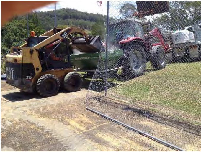
Plate 8 - Loading seed for revegetation works.
