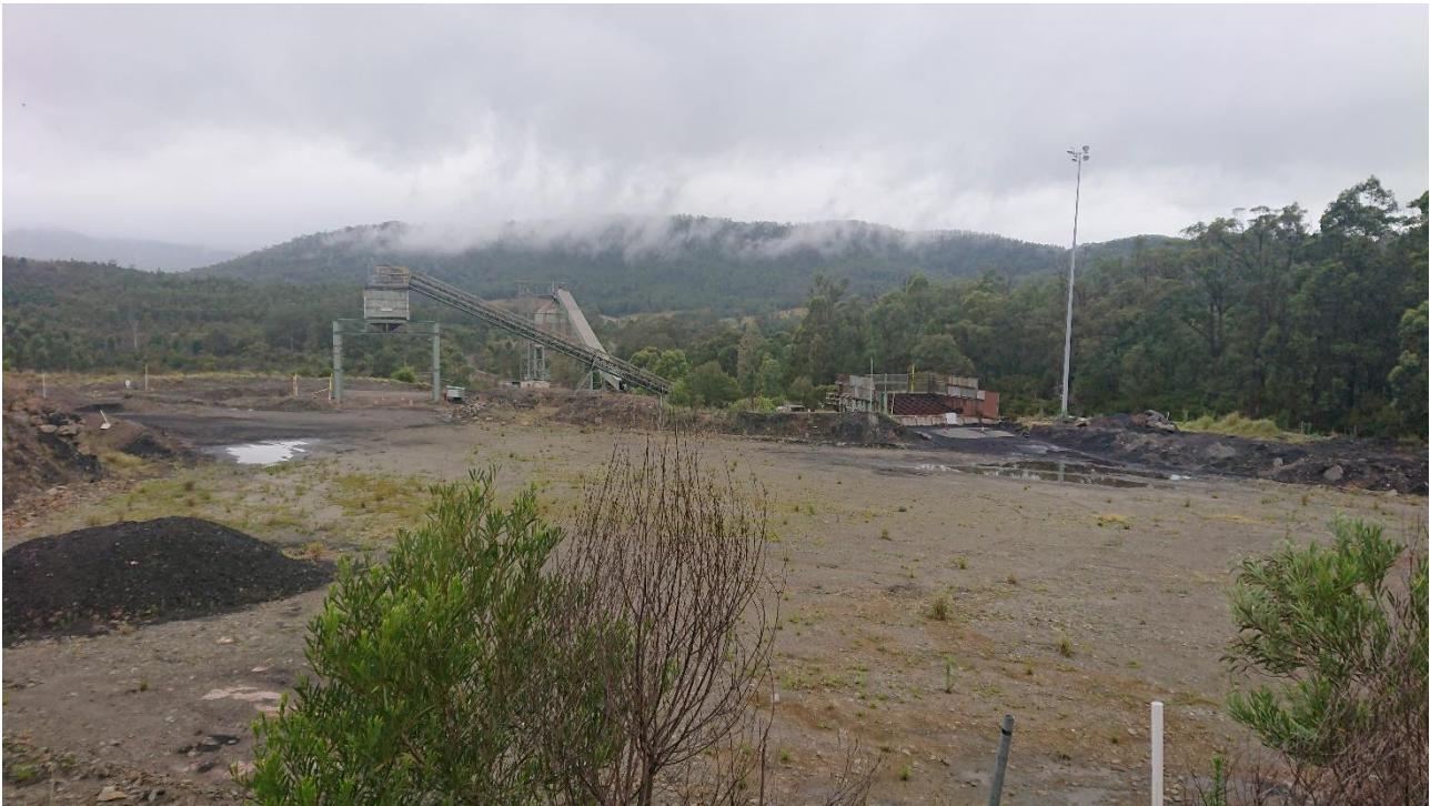
Photo 2 - Former ROM pad with rail loader in background
