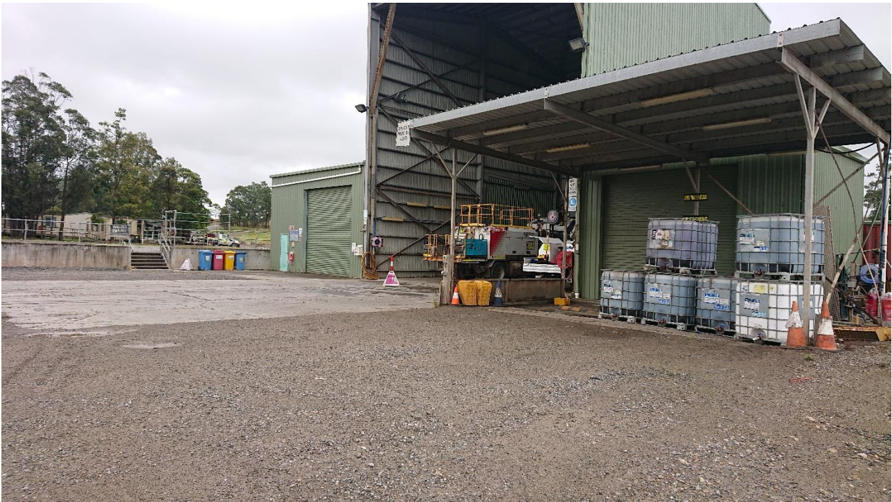
Photo 3 - Current Maintenance Area
