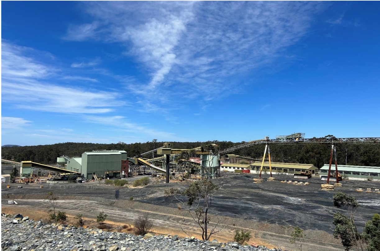
Plate 3 – ROM Coal Stockpile Area
