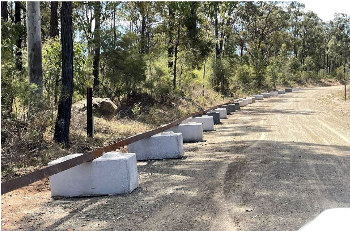
Plate 8 – Concrete barriers to restrict site access into previous mining, infrastructure and rehabilitated areas
