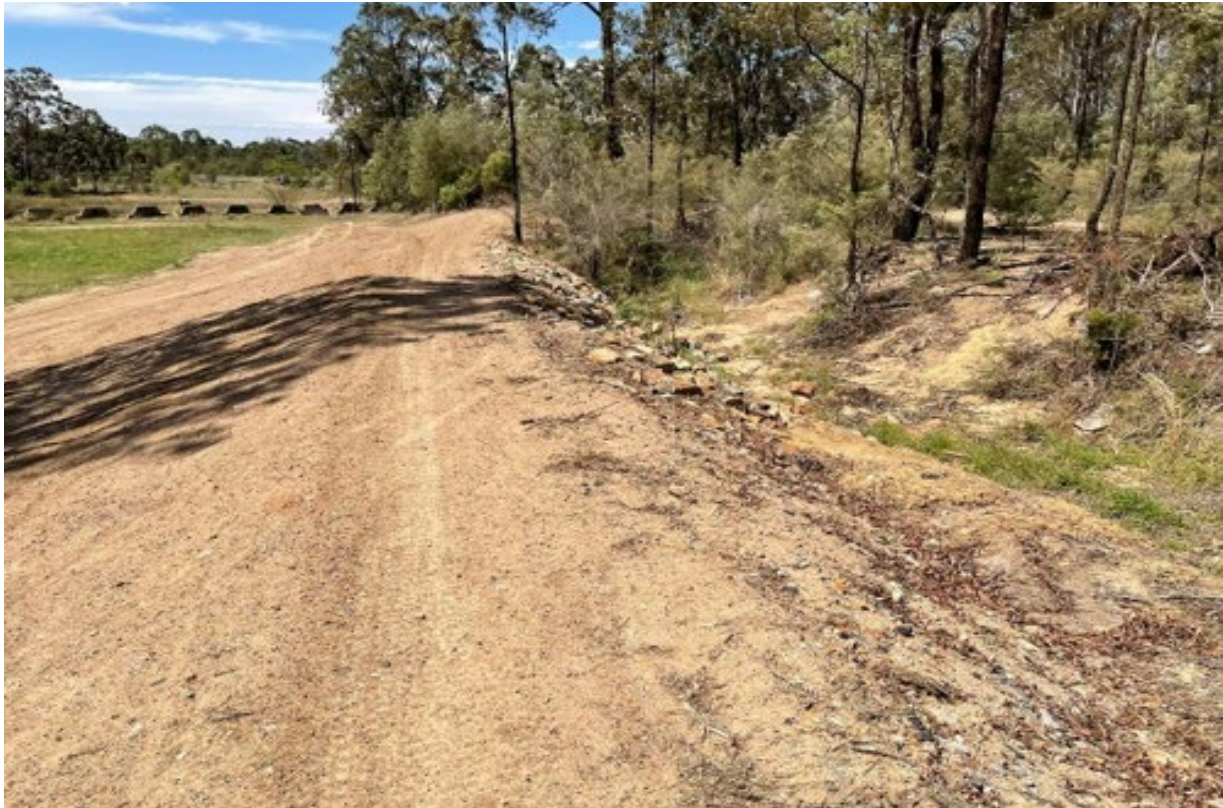
Plate 13 – Recently repaired clean water diversion drain awaiting hydroseeding
