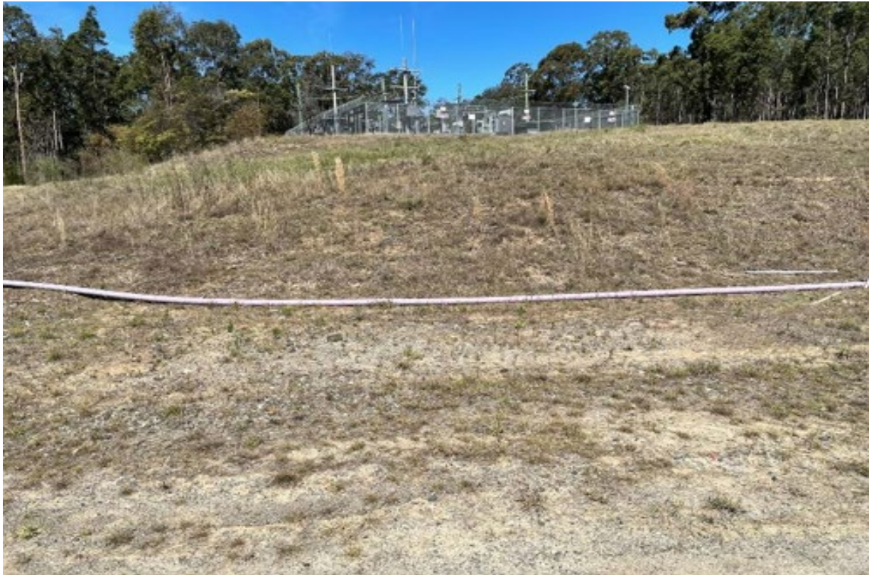
Plate 11 – Kitchener SIS with temporary rehabilitation on non-final land forms
