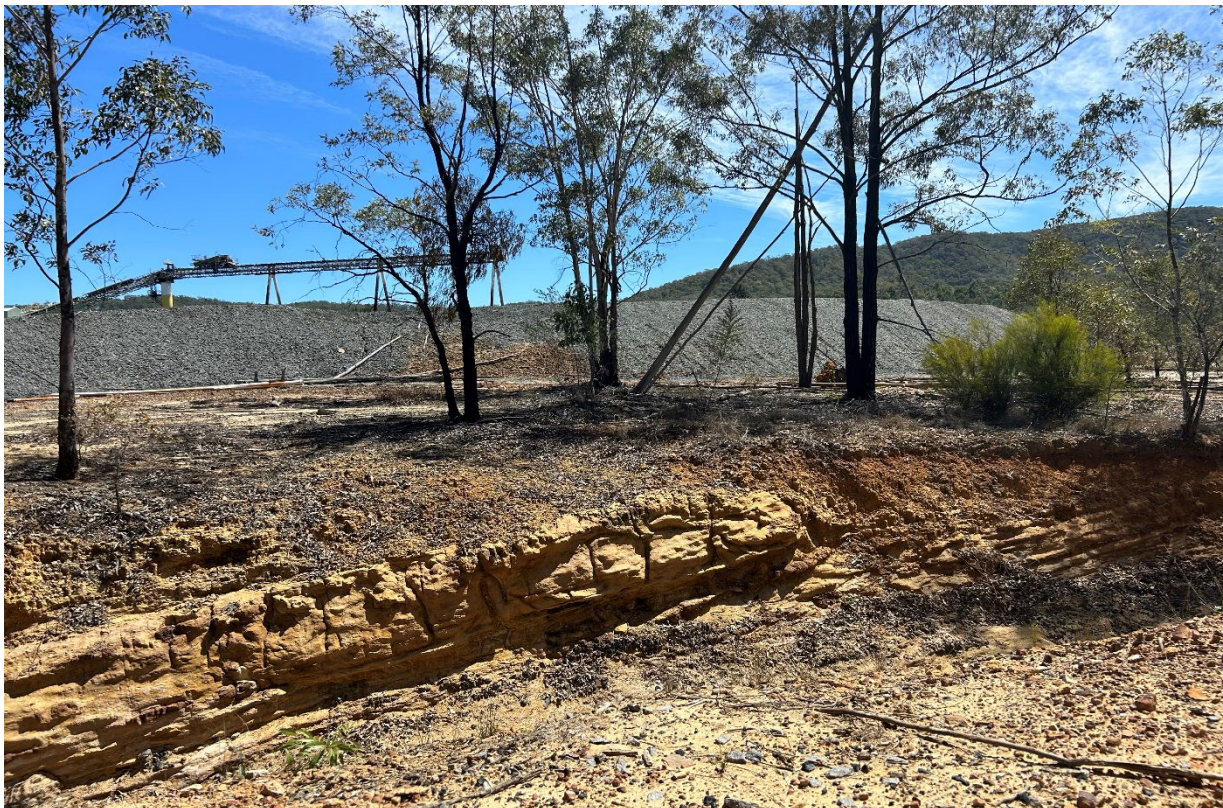
Plate 4 – Stockpile and drain directing runoff to water pollution control ponds
