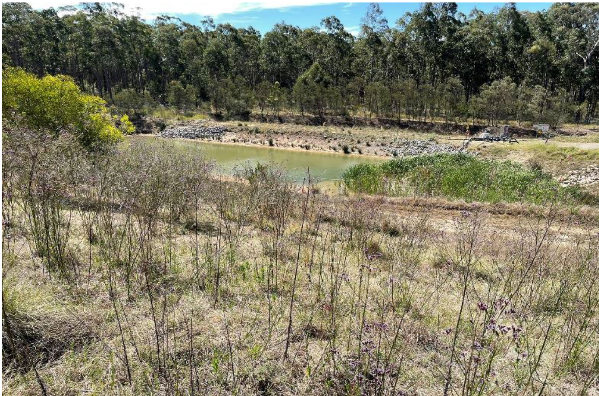
Plate 12 – Kitchener SIS surface water infrastructure
