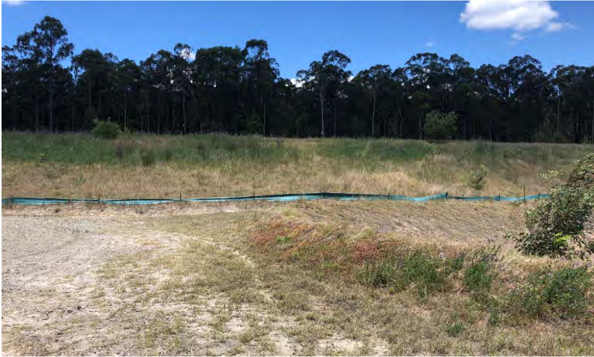
Photo 15 Possible consideration of clean water catchment at Kitchener SIS to reduce catchment reporting to the sediment dams. Successful rehabilitated area evident
