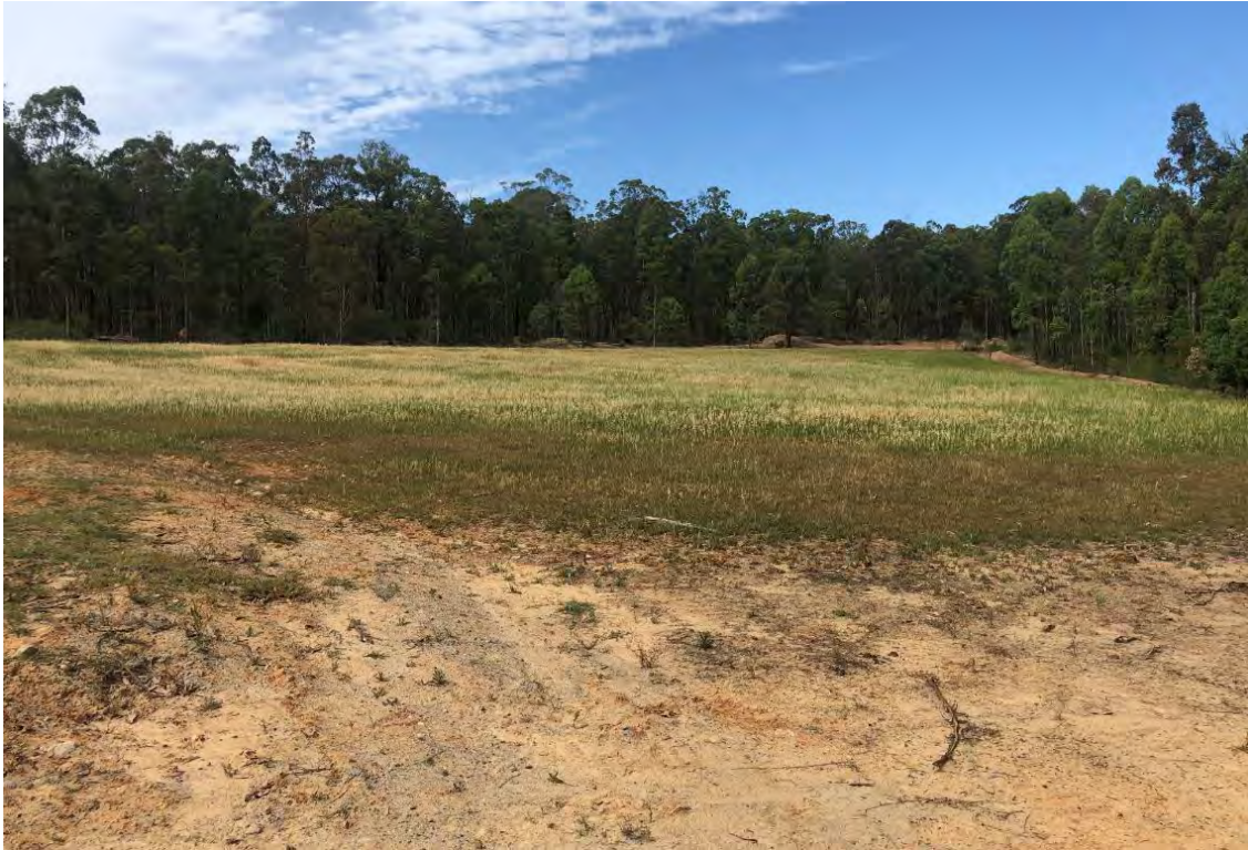
Photo 9 Success of cover and stability of rehab at West Pit Area
