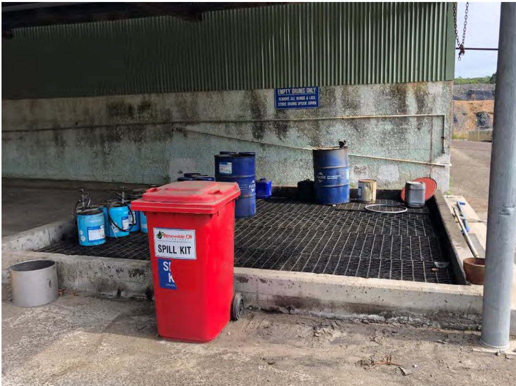
Photo 3 Generally good hydrocarbon management with containers in appropriately bunded areas
