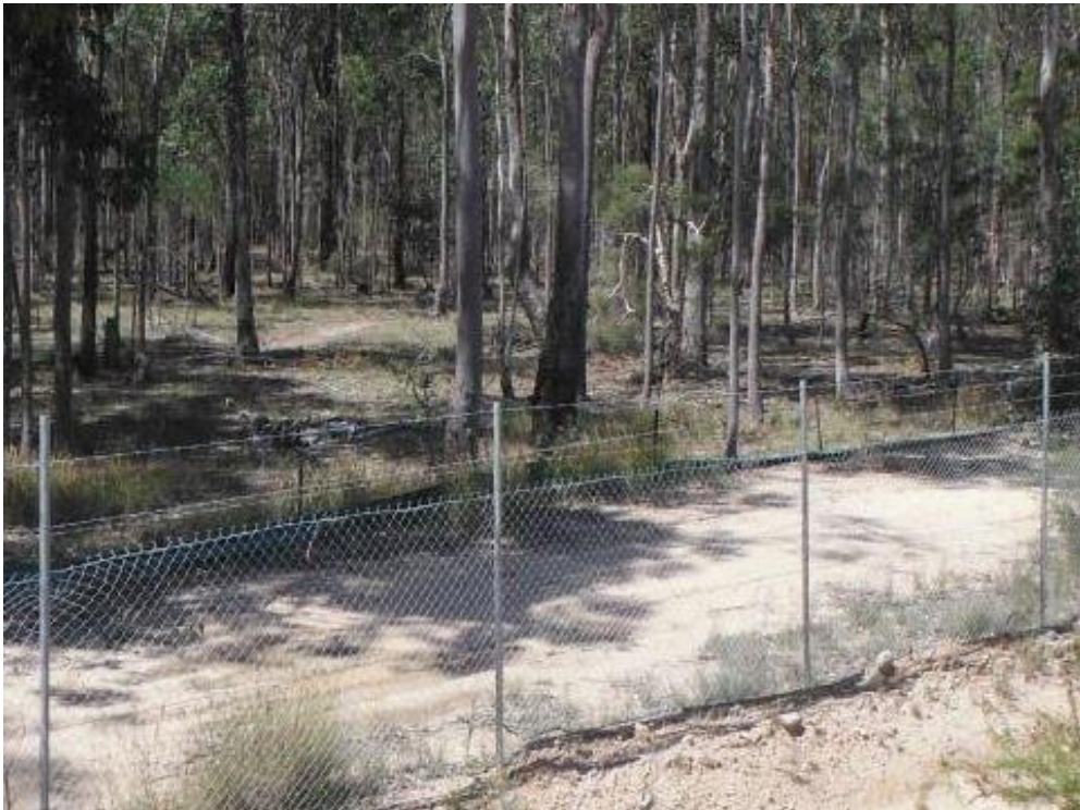
Photo 13 Evidence of erosion outside the boundary fence
