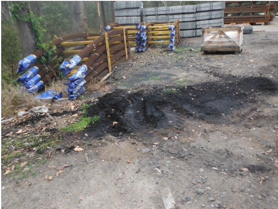
Photo 1 Small Amount of Coal Material at Laydown Area. To be removed
