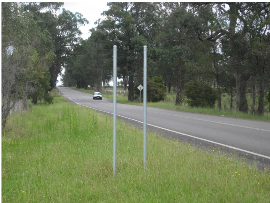
Photo 2 - Sandy Creek Road Condition in Bellbird South Mining Area (near Vandalised Subsidence Warning Sign posts)
