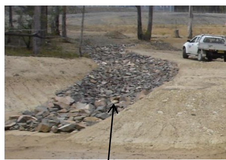
Rock lined channel into the western sediment basin
