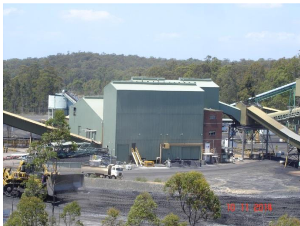
Plate 5.5.2.1: CHPP acoustic cladding on walls and roof.
