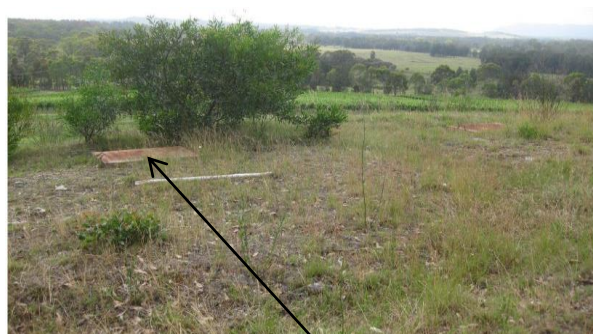
Plate 5.13.3b: Damaged in-ground tank location (steel plates) at Vineyard owned by Austar above Stage 2
