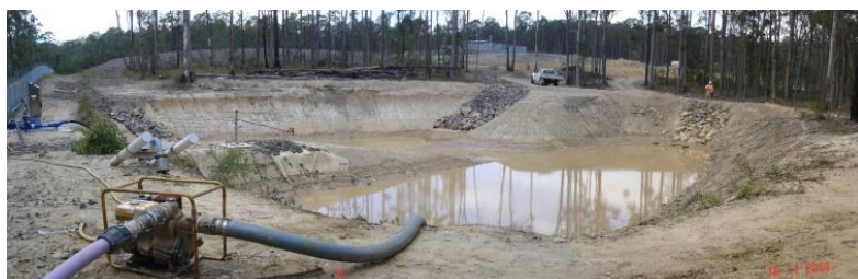
Western sediment basin east of the unnamed watercourse collecting runoff from the materials storage and handling area.
