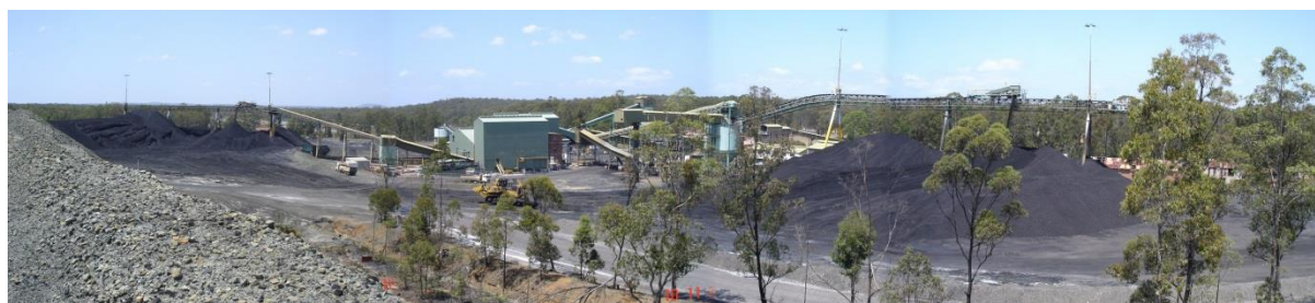
Plate 5.5.2.2: CHPP from the top of the noise bund between the CHPP refurbished building and receivers to the west and northwest
