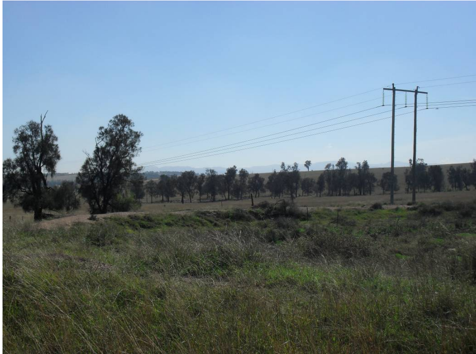
Figure 10: 2 pole power line and Dam
