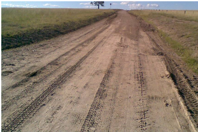
Figure 9: Access road post repairs.
