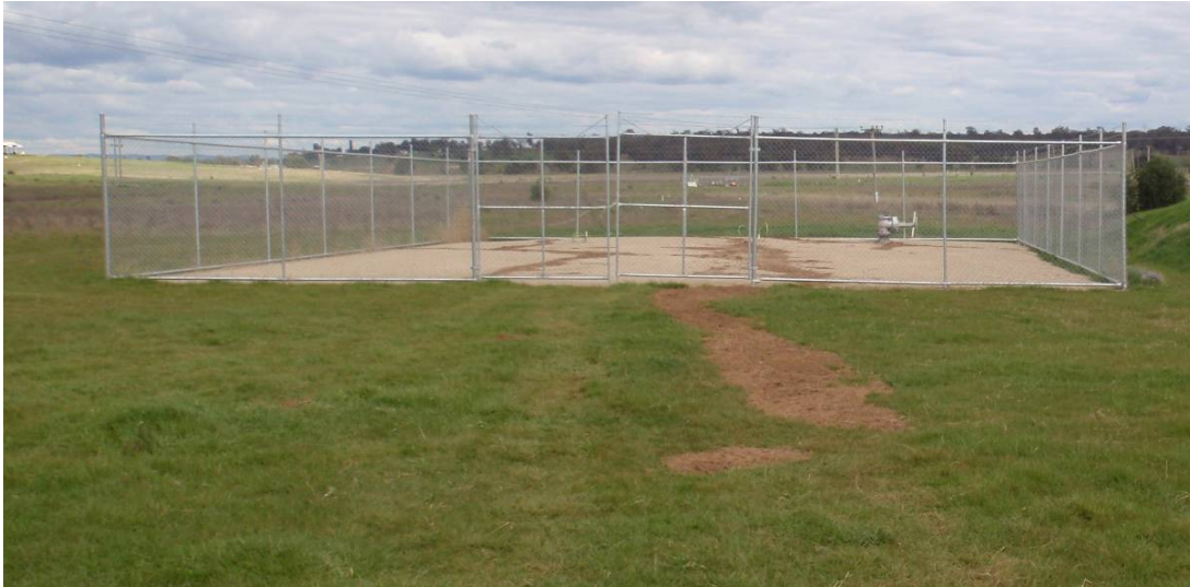
Figure 10: LW7A Gas drainage plant 5 following remediation (10/08/2011).
