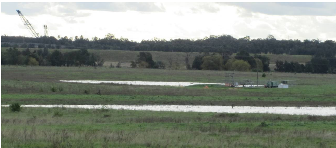
Figure 7: LW7A ponding in the background behind Gas Drainage Plant 4 (16/06/2011). The ponding in the foreground is dam 10 which includes the ponding caused by subsidence during Longwall 6A.
