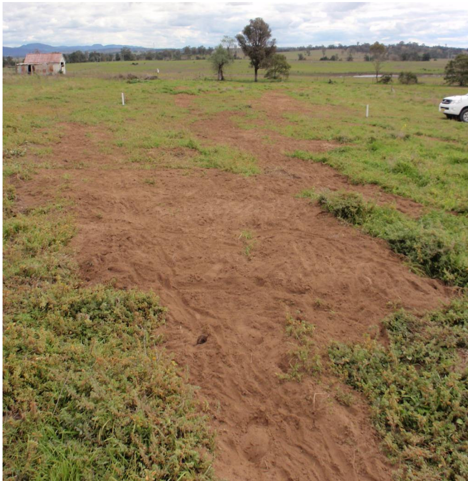
Figure 11: Longwall 5 secondary remediation (10/08/2011). Loam was used to re-level the ground following settling of the ripped soil.
